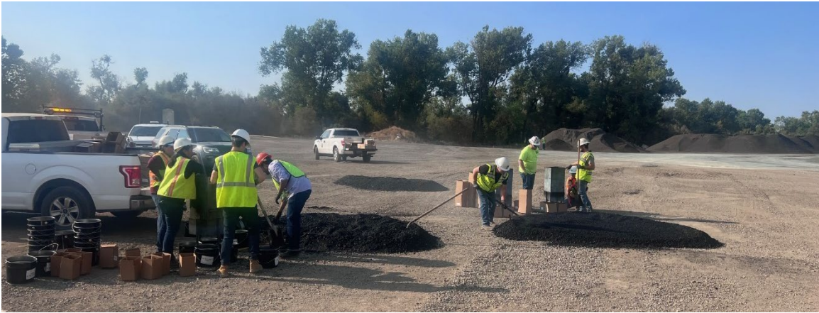
Figure 2.8: Sampling from hot drop and putting in buckets and boxes for QA sampling (each person is sampling from a quadrant of the pile of hot mix).
