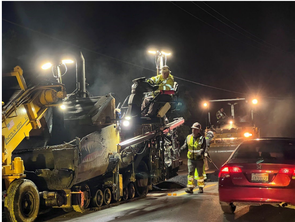
Figure 5.4: Mix laydown using a paving machine.
