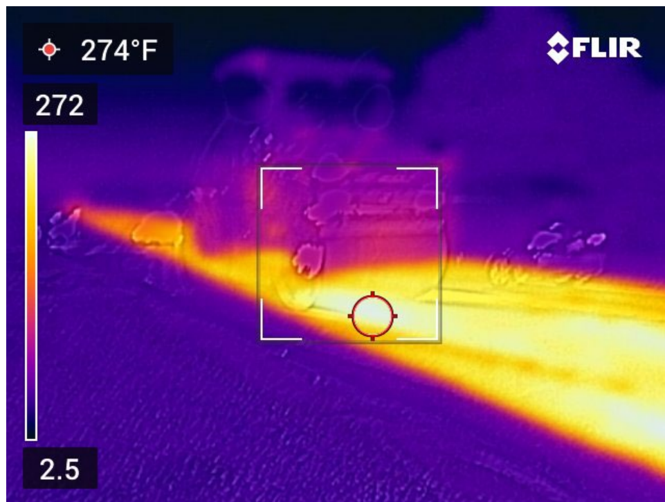
Figure 5.6: Thermal image of breakdown compaction of the mat on the high RAP and RAS sections.
