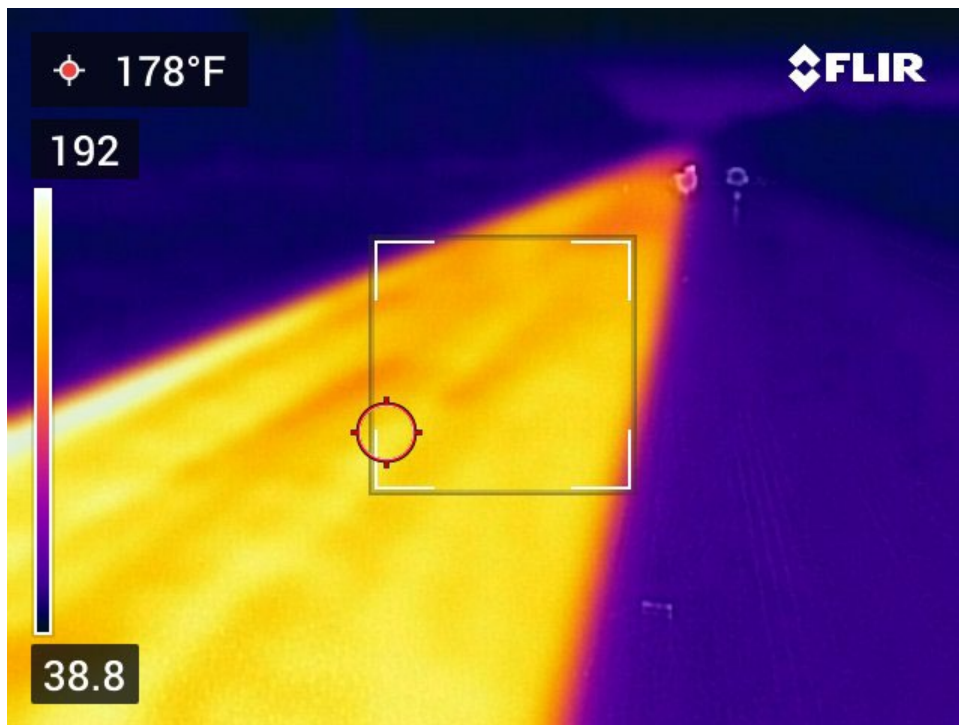
Figure 5.10: Thermal image of mat prior to final rolling and compaction on the high RAP and RAS sections.
