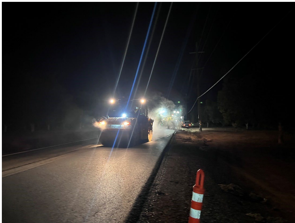
Figure 5.5: Breakdown compaction of the mat on the high RAP and RAS sections.
