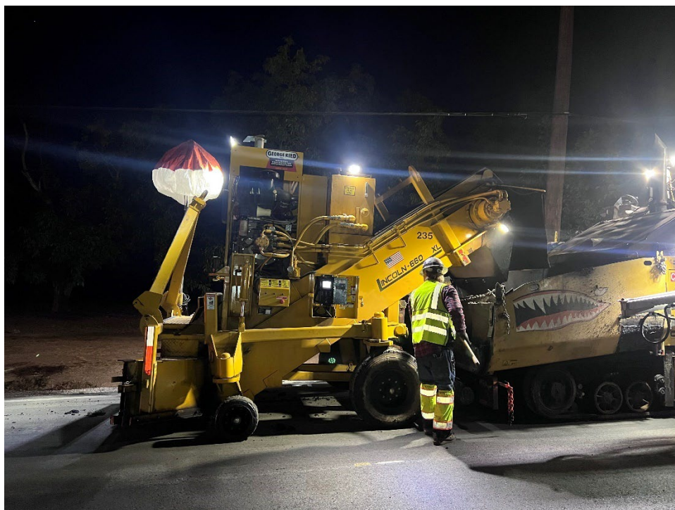
Figure 5.3: Windrow pick up using a material transfer vehicle.
