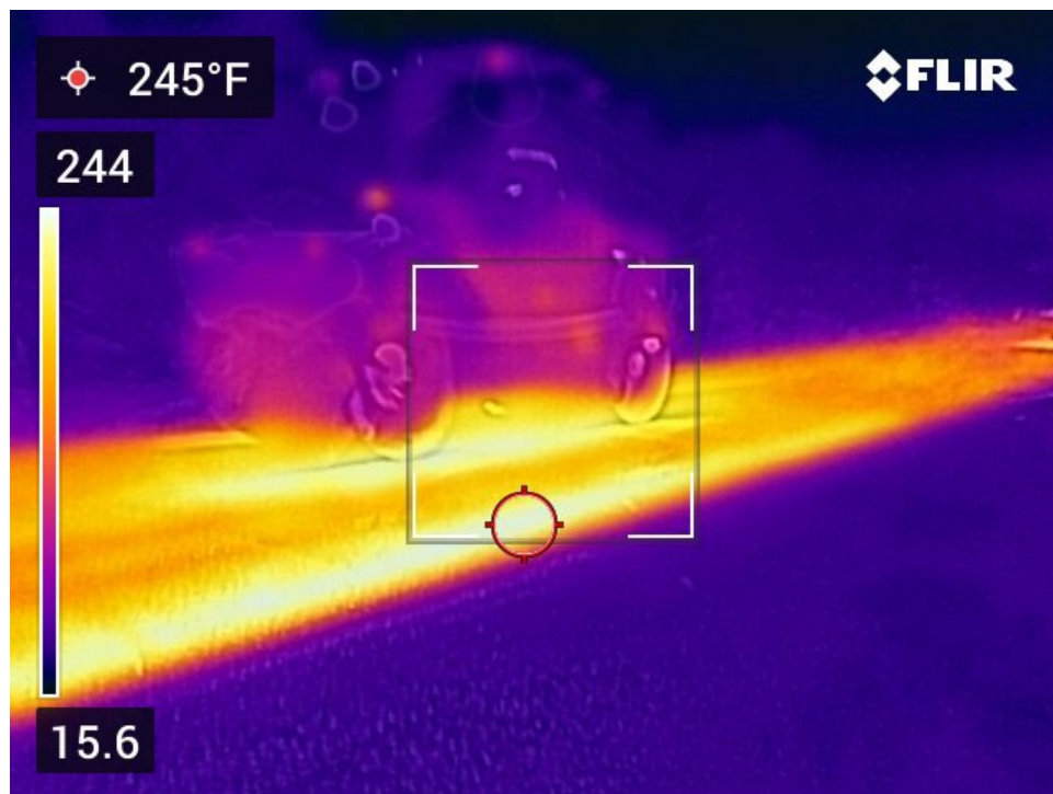
Figure 5.8: Thermal image of intermediate compaction of the mat on the high RAP and RAS sections.
