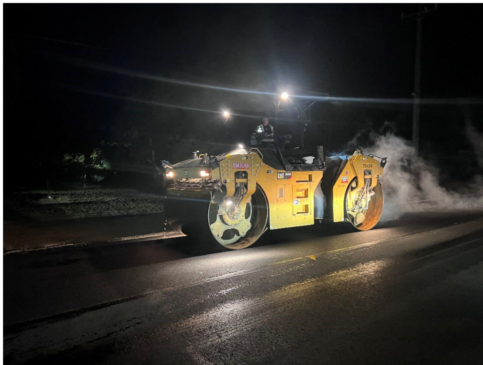
Figure 5.7: Intermediate compaction of the mat on the high RAP and RAS sections.
