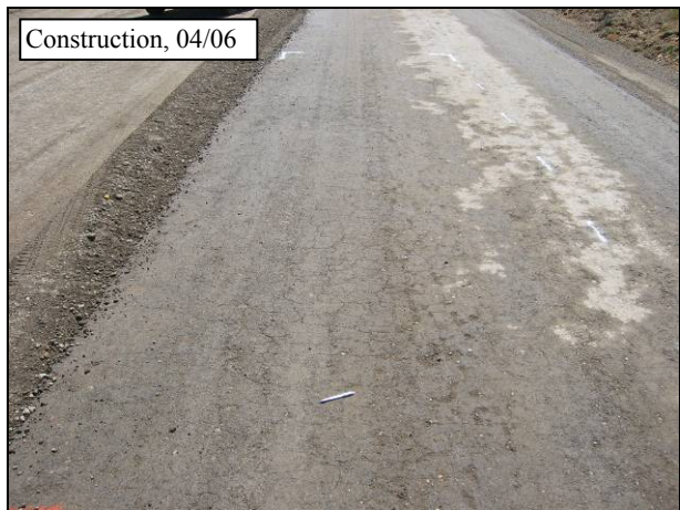
Figure 4.55: Area demarcated for rework on 07-VEN-33.
