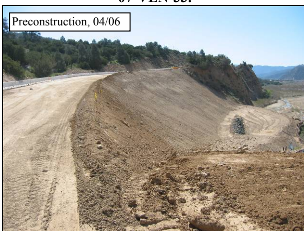
Figure 4.40: Pre-construction landslide repair on 07-VEN-33.
