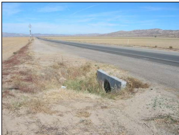
Figure 4.18: Filled in side drains on 05-SB,SLO-33.
