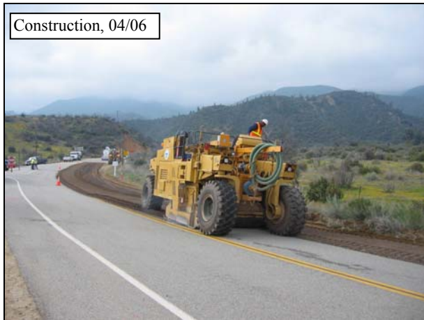
Figure 4.43: Prepulverization on on 07-VEN-33.
