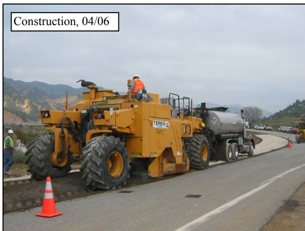
Figure 4.45: Foamed asphalt injection (Train 1) on 07-VEN-33.
