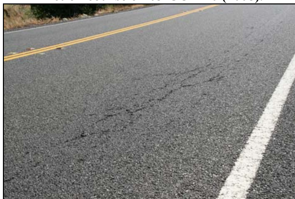
Figure 4.6: Longitudinal cracks in hill section on 03-COL-20 (2007–2008).
