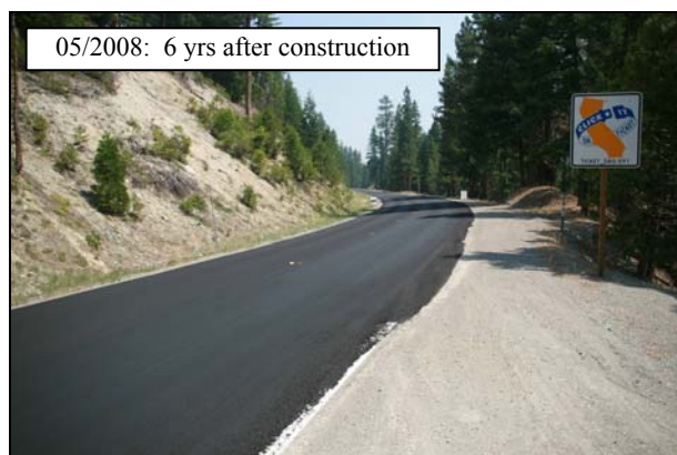
Figure 4.11: Pavement preservation treatment on 03-SIE-89.
