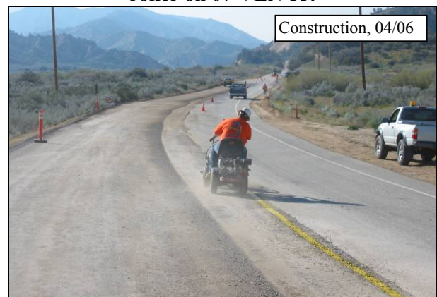
Figure 4.52: Temporary striping application on 07-VEN-33.
