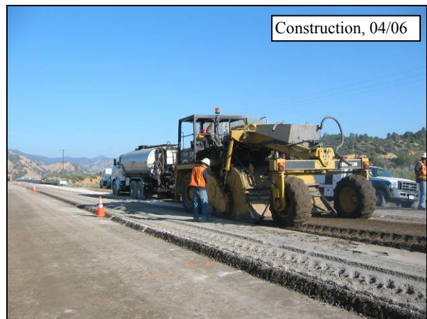
Figure 4.46: Foamed asphalt injection (Train 2) on 07-VEN-33.
