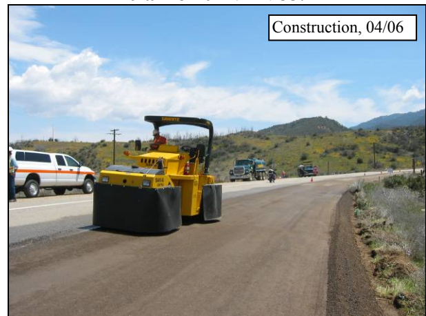
Figure 4.50: Final compaction with rubber-tired roller on 07-VEN-33.
