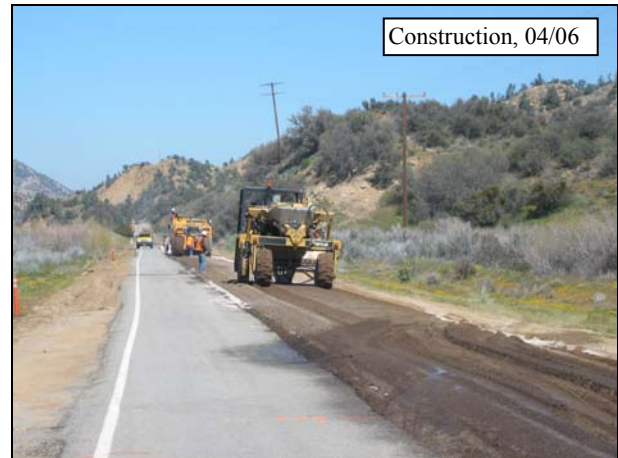
Figure 4.48: Water application behind recycling train on 07-VEN-33.
