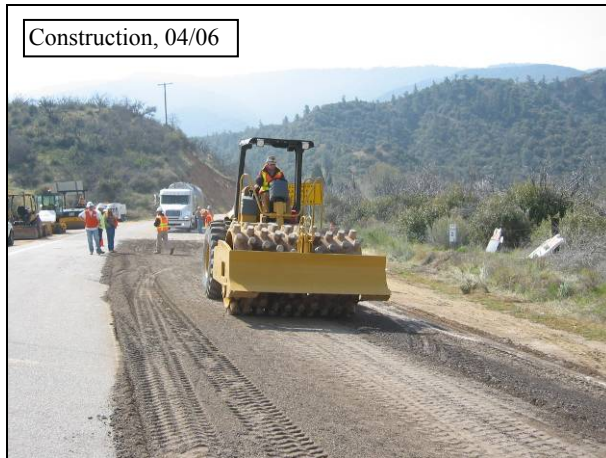
Figure 4.47: Initial compaction with padfoot roller on 07-VEN-33.
