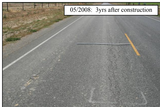
Figure 4.26: New areas of distress on 05-SB,SLO-33 (May 2008).
