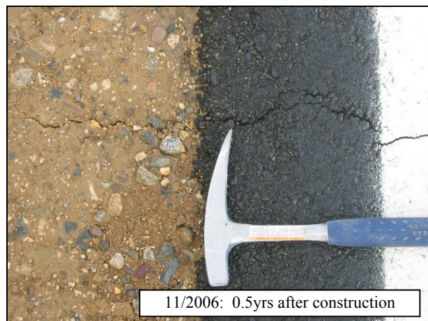
Figure 4.58: Transverse cracking on 07-VEN-33.
