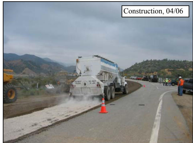
Figure 4.44: Cement kiln dust application on 07-VEN-33.
