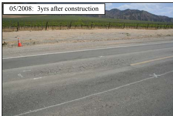
Figure 4.26: New areas of distress on 05-SB,SLO-33 (May 2008).
