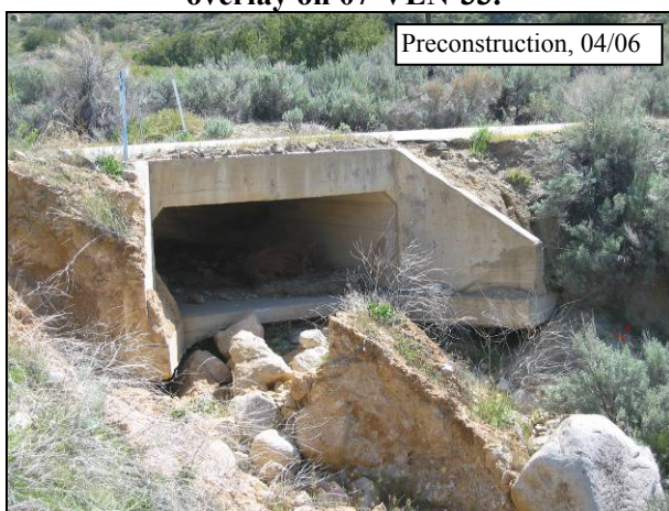
Figure 4.41: Drainage structure on 07-VEN-33.
