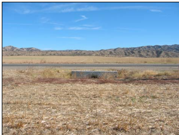
Figure 4.18: Filled in side drains on 05-SB,SLO-33.
