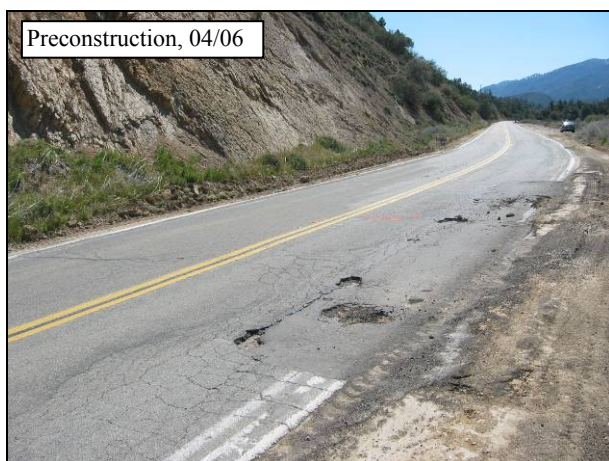
Figure 4.38: Preconstruction patching on 07-VEN-33.
