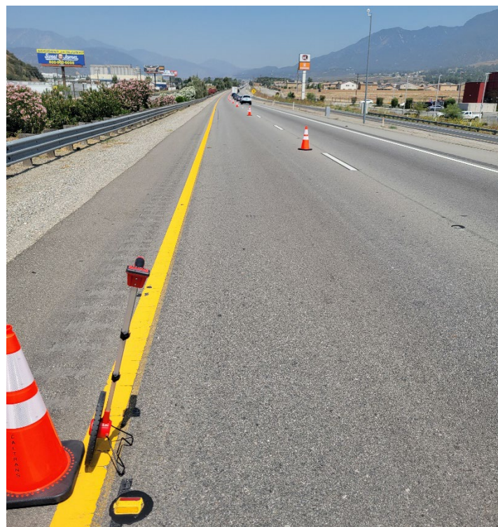
Figure 3.7. SBD 215 northbound at PM 14.20 (start of the 35% RAP mix).
