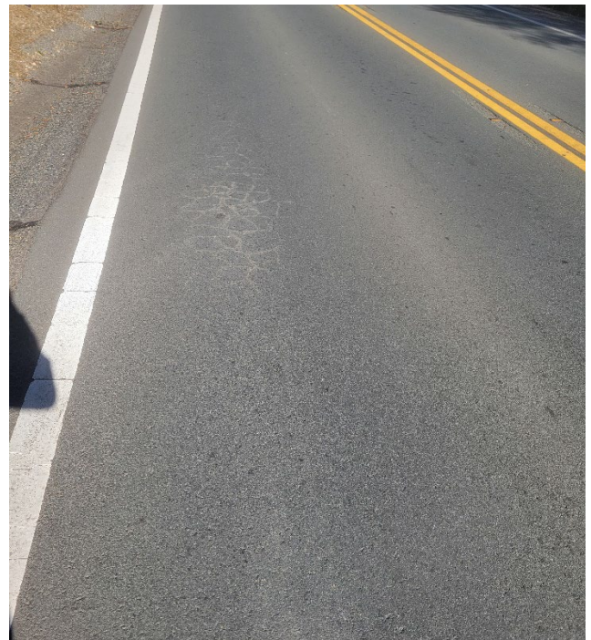
Figure 3.2. Alligator cracking with mild pumping (evident throughout project).
