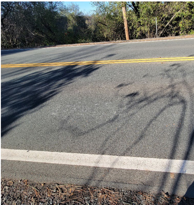
Figure 3.2. Alligator cracking with mild pumping (evident throughout project).
