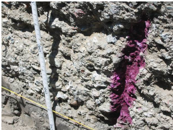
Figure 3.68: 591RF strongly cemented base.
