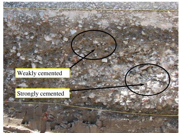
Figure 3.41: 587RF#12 areas of strong and weak base cementation.
