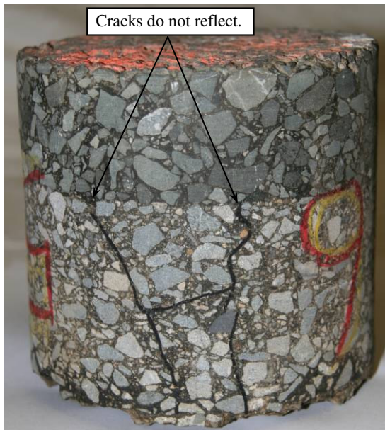
Figure 3.70: MB15-G: Cracks on core.
