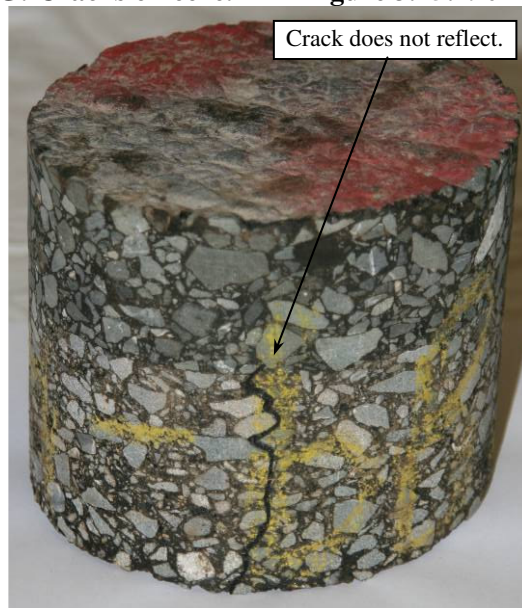
Figure 3.76: MAC15-G: Cracks on core.
