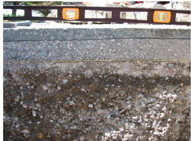
Figure 3.39: 587RF#12 absence of visible cracks.
