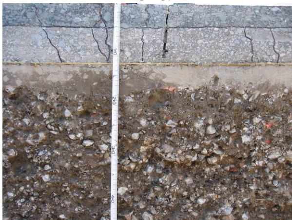
Figure 3.40: 587RF#4 weaker cemented base material.
