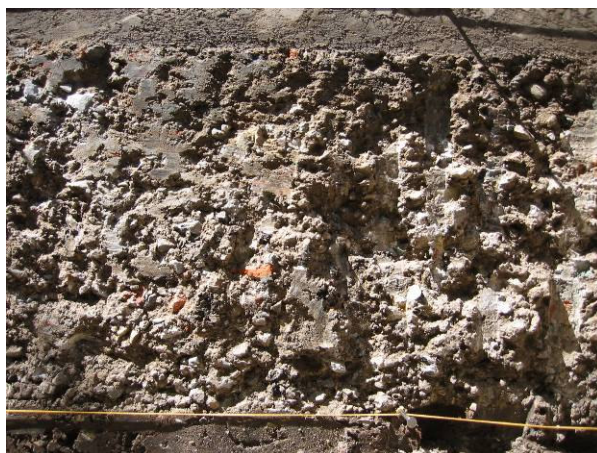
Figure 3.33: 586RF strongly cemented base.
