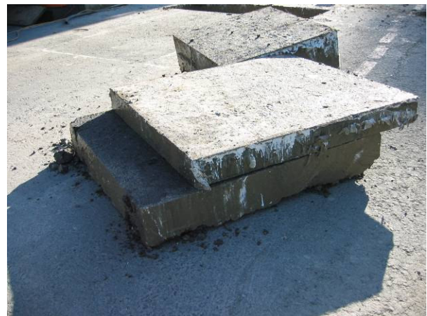
Figure 3.45: 588RF debonding between overlay and underlying layer.
