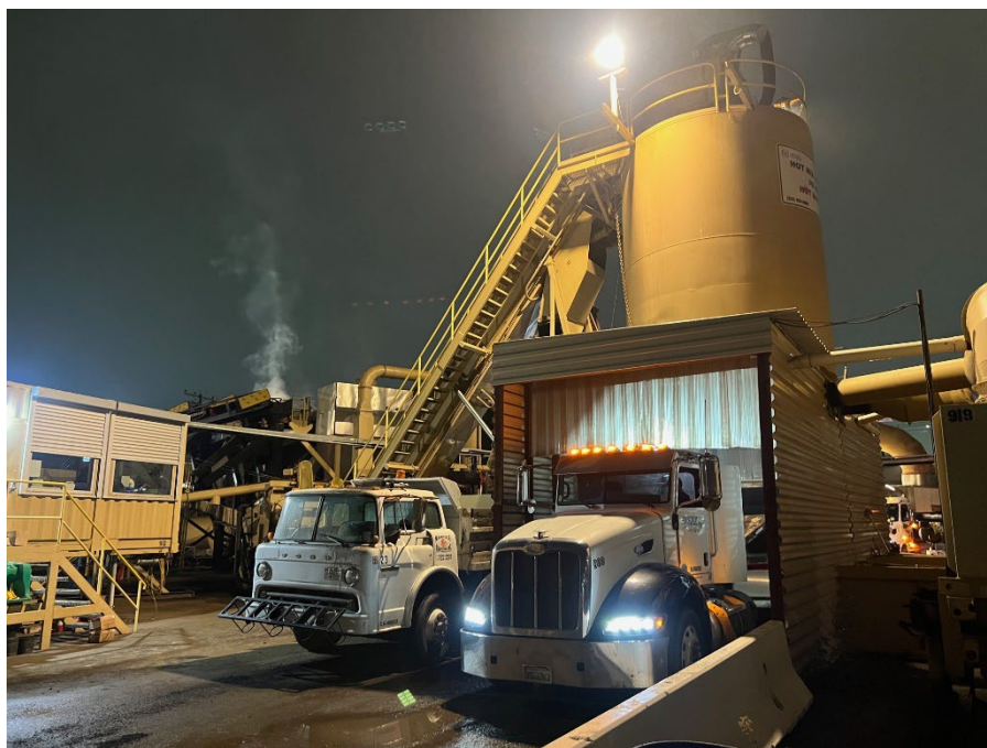
Figure 2.5: Truck load out at the HyRAP mixing plant (also the point of sampling).
