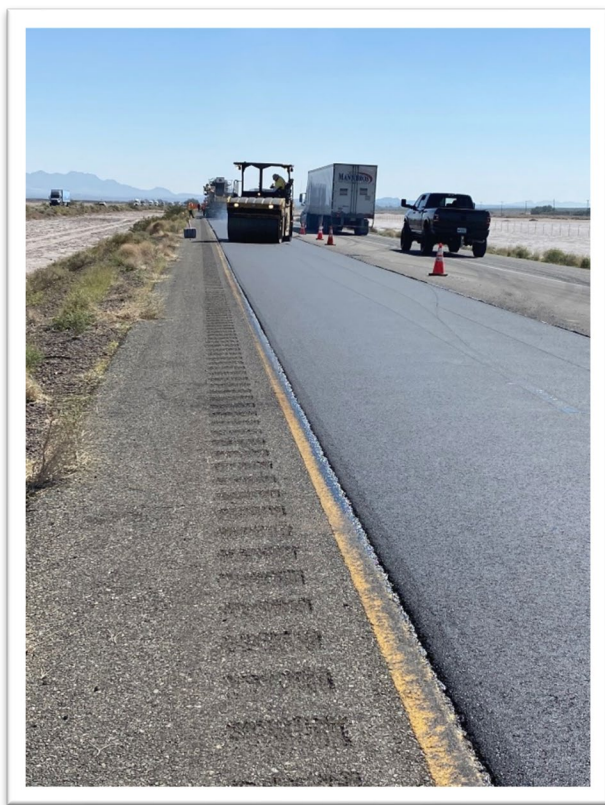
Figure 1 – HyRAP paving operation
