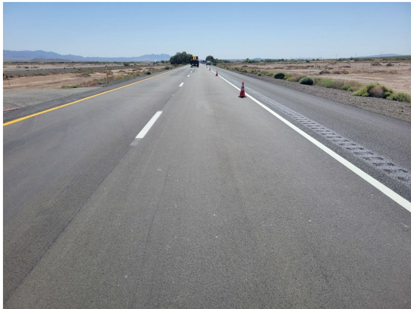
Figure 3.3: Completed HyRAP 100% RAP material mat.
