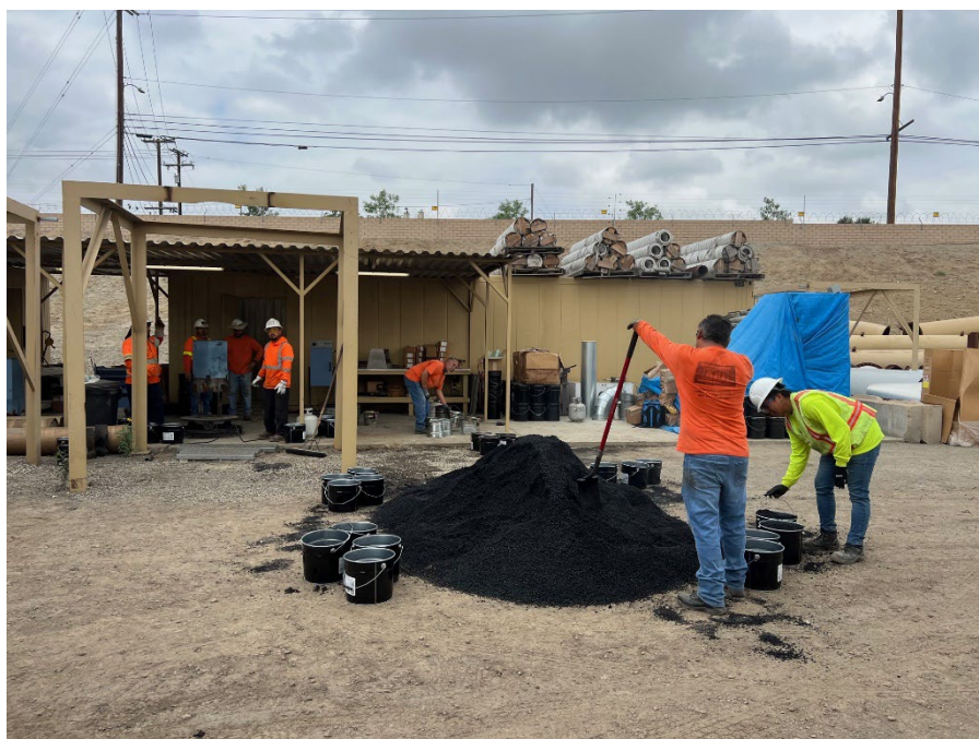
Figure 2.6: Quarterming and sampling of hot mix.
