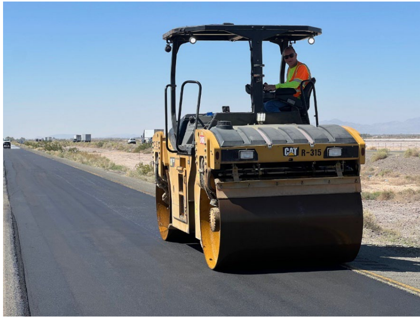
Figure 3.2: Static steel rolling on HyRAP 100% RAP material.
