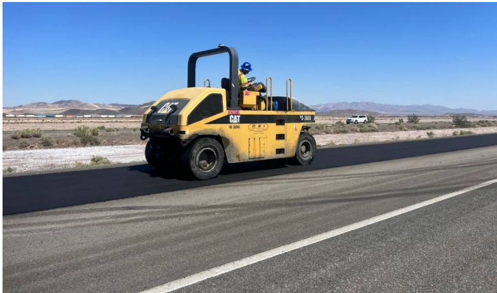
Figure 3.1: Pneumatic tire rolling on HyRAP 100% RAP material.
