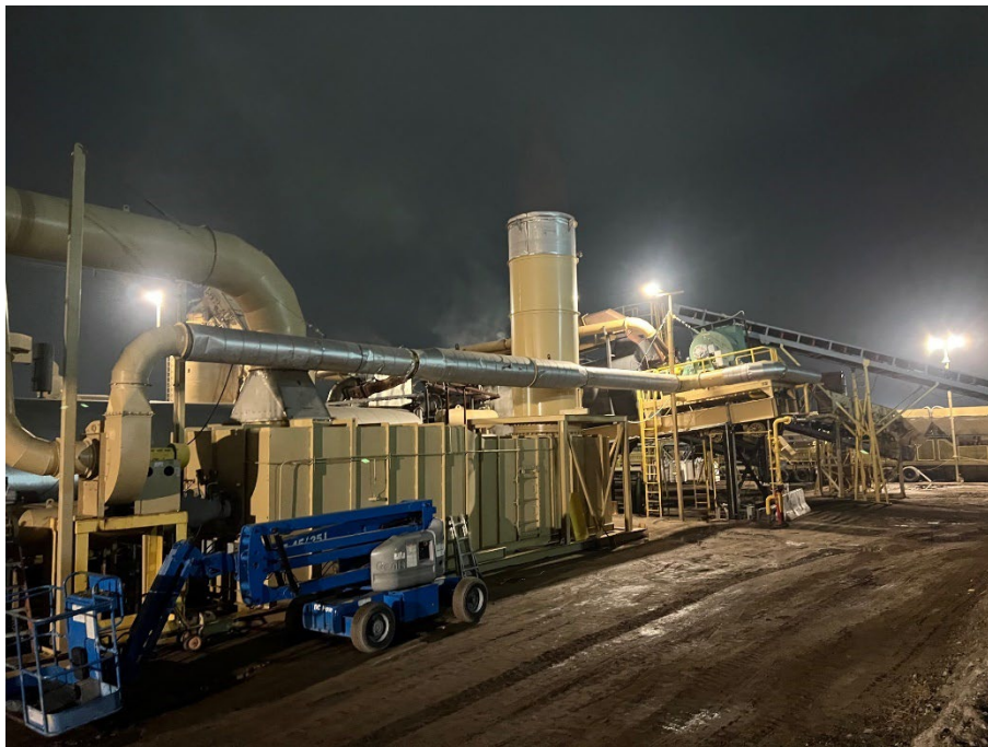
Figure 2.4: Oxidizer for burning volatile emissions.
