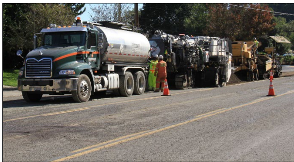
Figure 6.6: Single-unit PDR recycling train.
