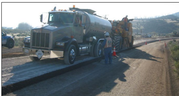
Figure 6.75: FDR-FA recycling train with no water tanker.
