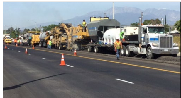
Figure 6.7: Multi-unit PDR recycling train.
