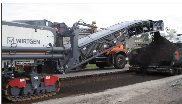
Figure 6.79: PDR project with belt feed into paver.
