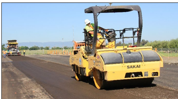
Figure 6.13: Steel breakdown roller on a PDR layer.
