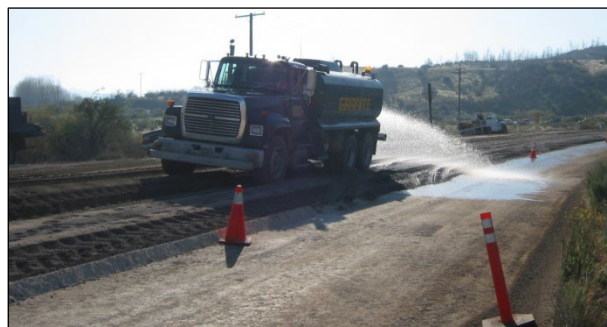
Figure 6.76: Separate water application behind recycler (FDR).
