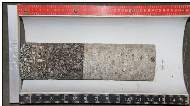
Figure 2.43: Concrete beneath asphalt layers (composite pavement).
