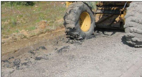
Figure 6.41: Effect of problem nozzles on an FDR-FA project.
