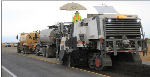
Figure 1.2: Partial-depth recycling train (single unit).
