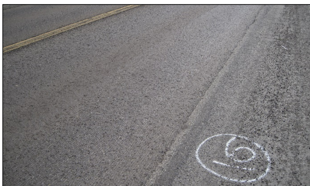
Figure 6.119: PDR layer milled for smoothness prior to placing asphalt concrete surface.
