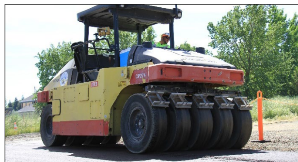
Figure 6.14: Pneumatic-tired roller on a PDR layer.
