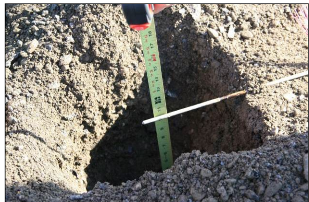
Figure 6.28: Checking recycling depth in a hole on an FDR project.
