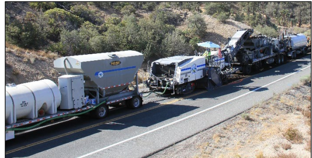
Figure 1.3: Partial-depth recycling train (multi-unit).
