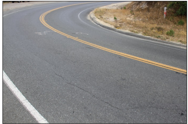
Figure 4.3: Point Arena Evotherm, November 2010, showing longitudinal cracks.
