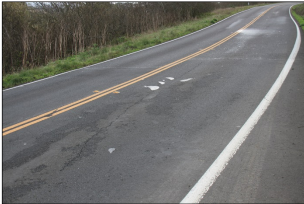
Figure 4.3: Point Arena Evotherm, November 2010, showing longitudinal cracks.
