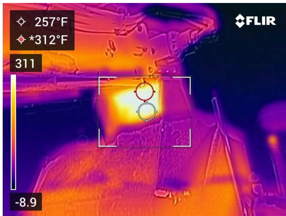
Figure 5.7: Mix exiting the shuttle buggy to the hopper of the paver.
