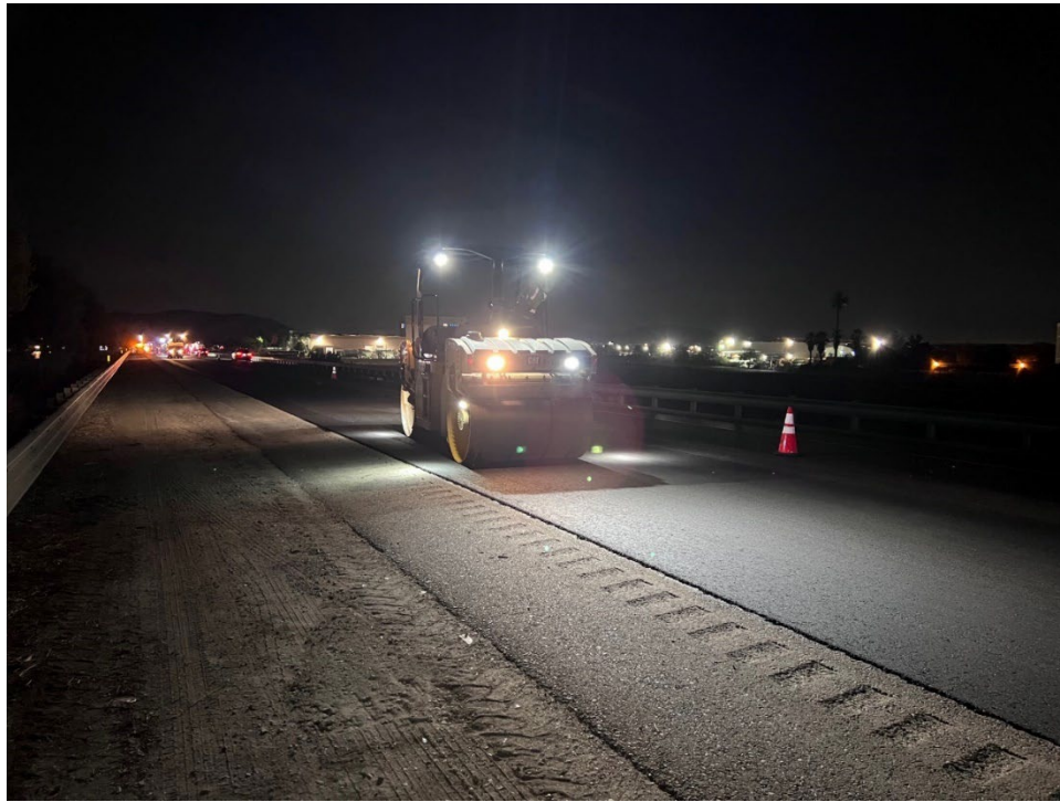
Figure 5.14: Finish roller.
