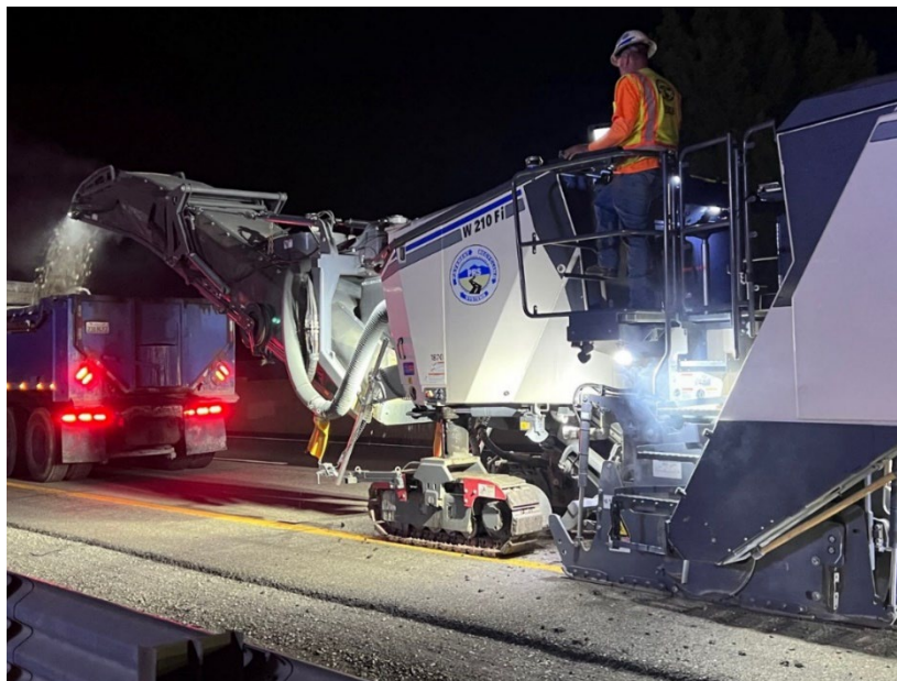
Figure 5.1: Milling operation.
