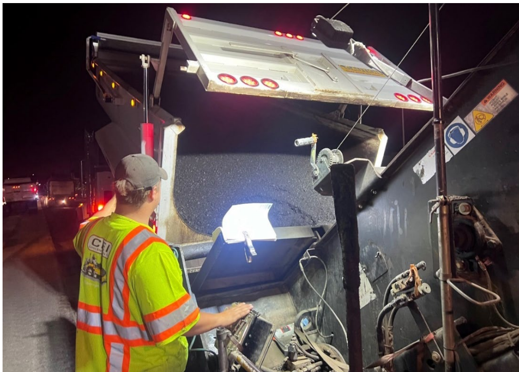
Figure 5.5: Placement of material from transfer to shuttle buggy.
