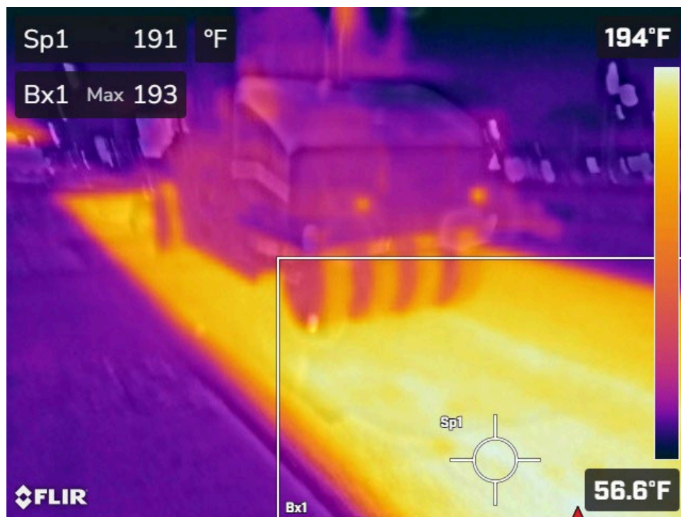
Figure 5.13: Thermal image of mat under intermediate pneumatic-tired roller compaction.
