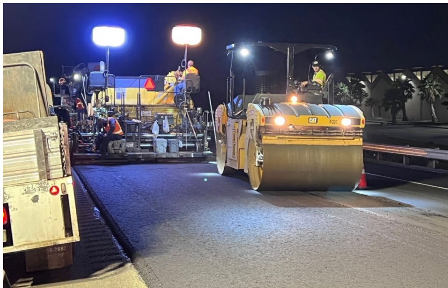
Figure 5.9: Breakdown roller.
