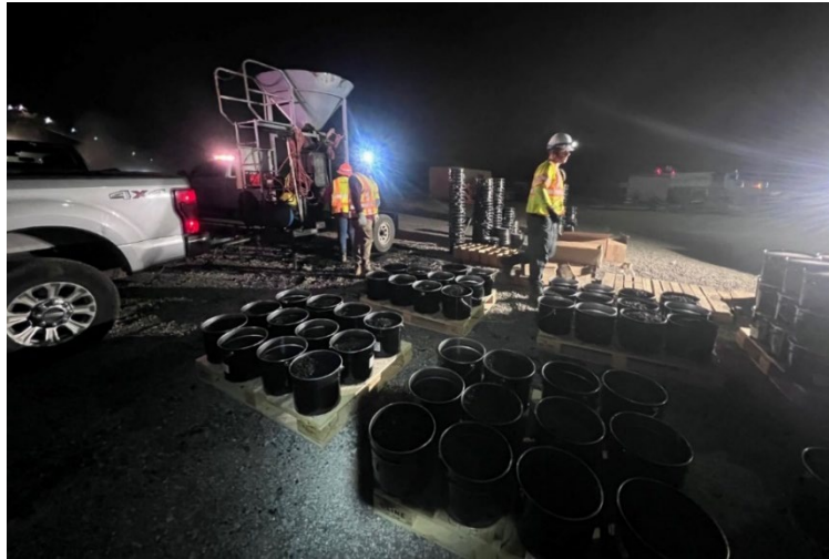
Figure 2.11: Sampling from hot drop and placement in buckets and boxes for quality assurance (QA) sampling on SBD 215.
