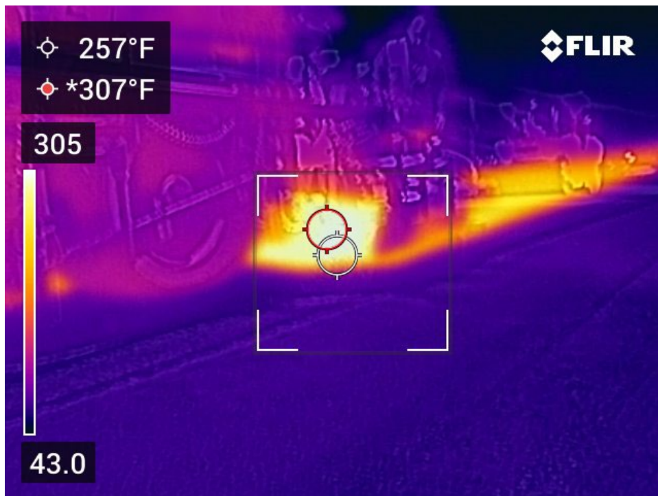
Figure 5.8: Mix feeding through the paver auger to the screed.
