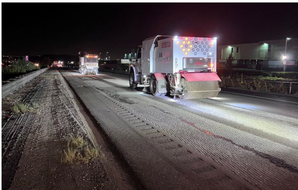
Figure 5.2: Sweeping prior to tacking and paving.
