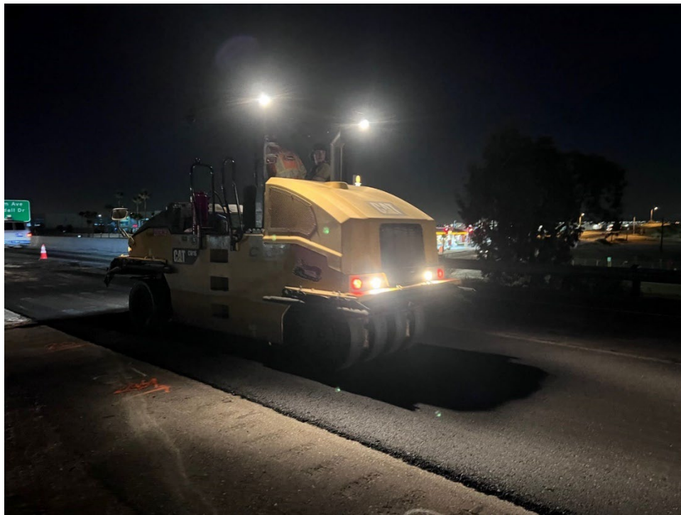
Figure 5.12: Pneumatic-tired intermediate roller.
