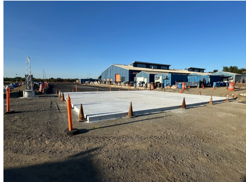
Figure 3.17: JPCP after construction.
