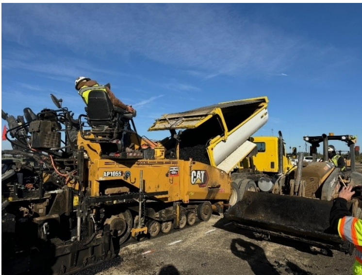
Figure 5.2: Asphalt paver and truck on primed aggregate base.
