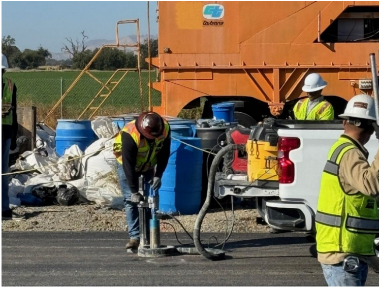
Figure 5.9: Coring on Lane 1.
