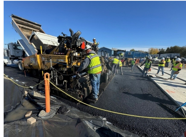
Figure 5.3: Intermediate layer lift 1 (0.2 ft.) paving.
