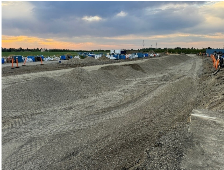
Figure 3.11: Imported Class II aggregate base before construction.
