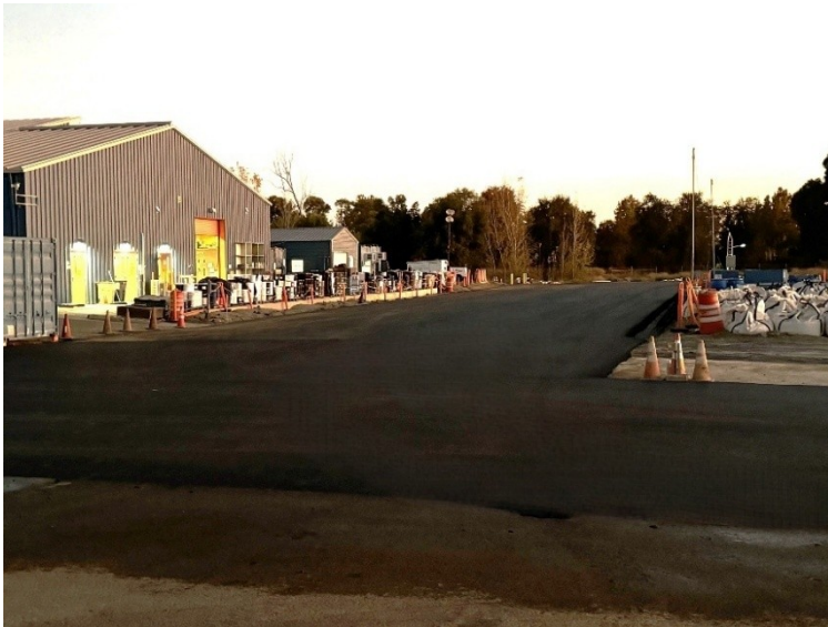
Figure 5.10: Test track after construction.
