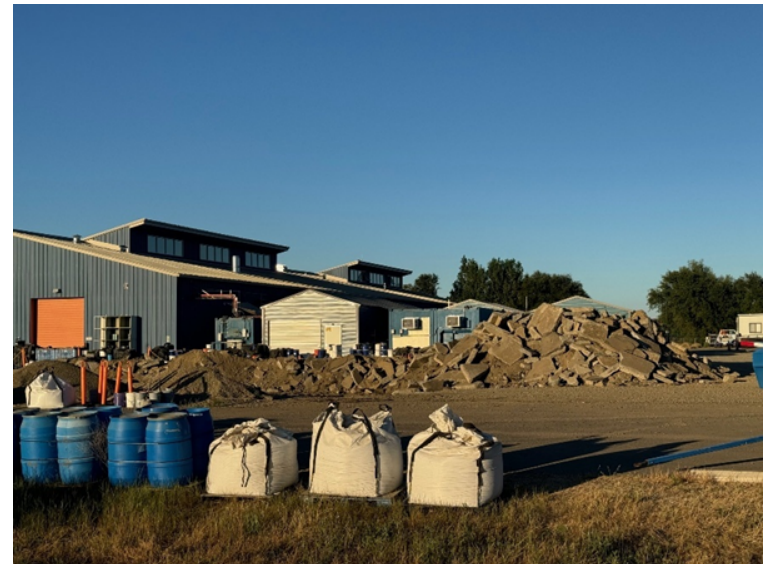
Figure 3.5: Stockpile of removed concrete pavement.
