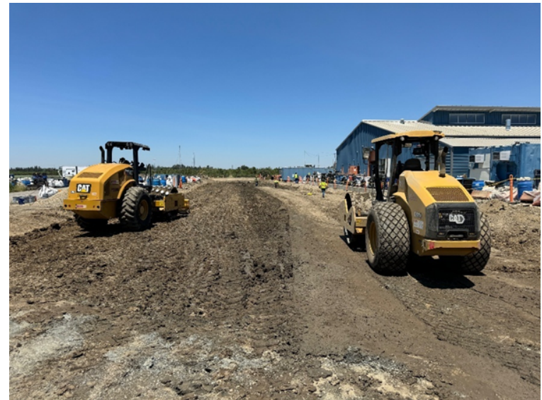
Figure 3.9: Subgrade recompaction.
