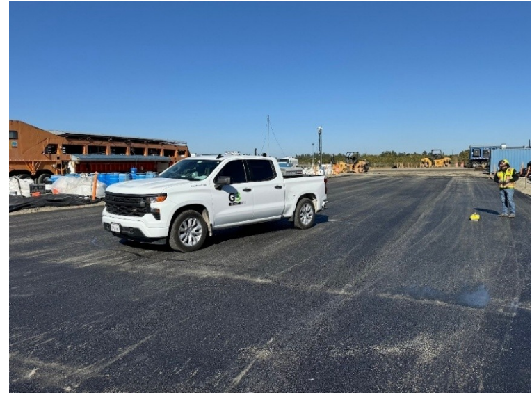
Figure 5.7: Nuclear gauge testing.
