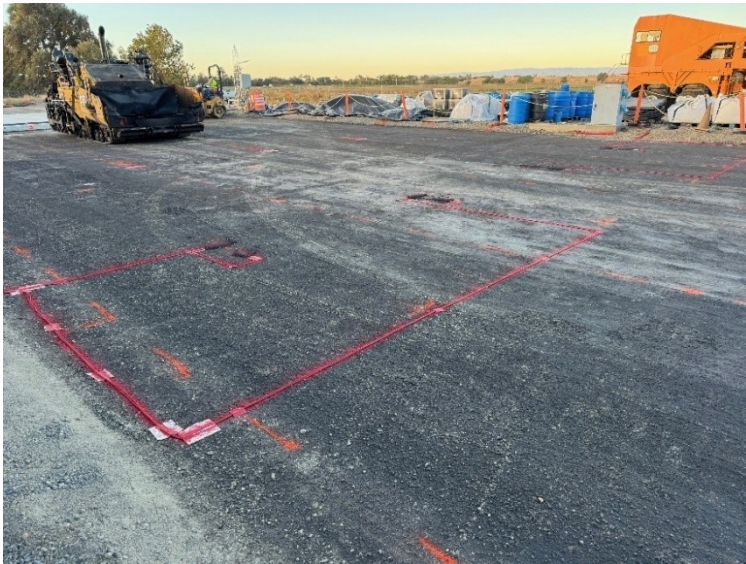
Figure 5.1: Instrumentation on primed aggregate base.
