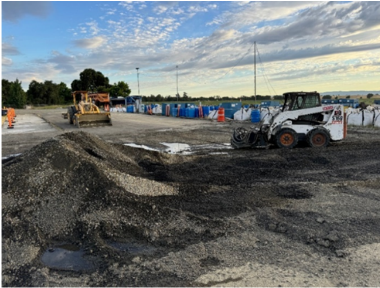
Figure 3.2: Milling of existing asphalt pavement.
