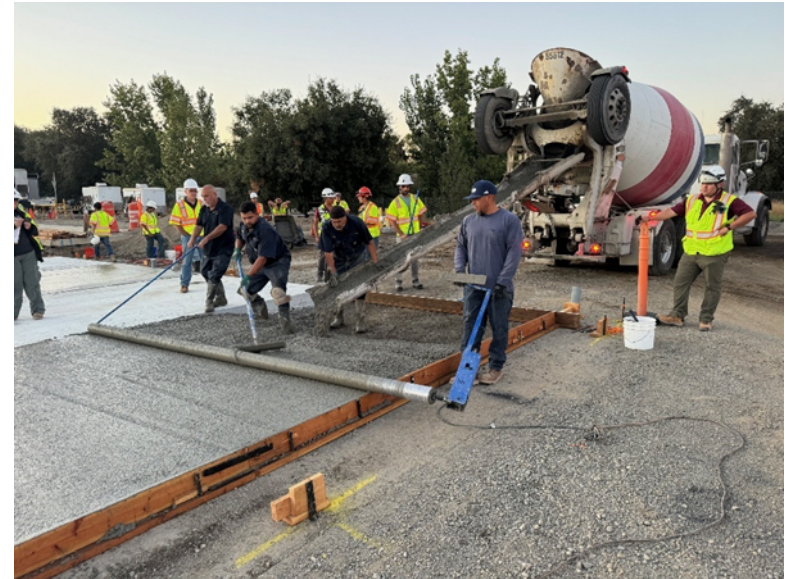
Figure 3.16: PCC placement.
