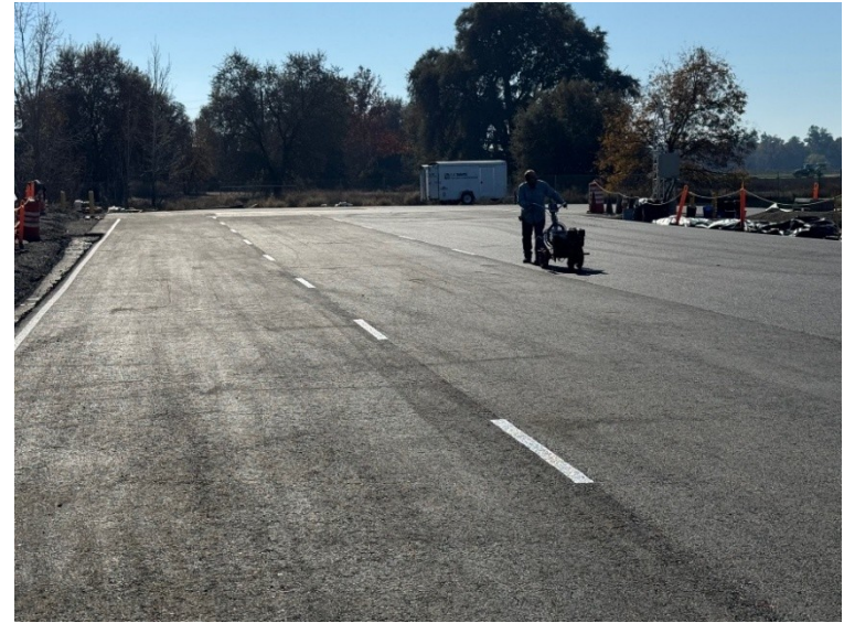
Figure 5.11: Line striping on test track.
