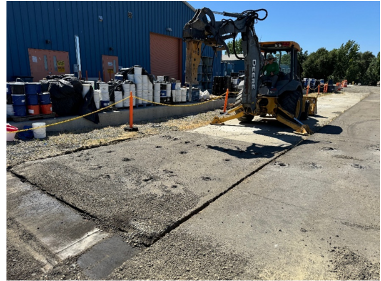
Figure 3.3: Breaking concrete with jackhammer.
