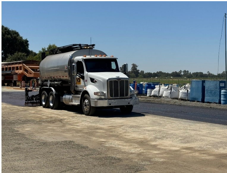
Figure 3.33: Prime coat placement on the aggregate base.
