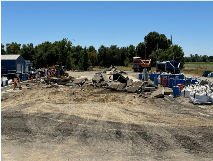
Figure 3.6: Demolished JPCP.
