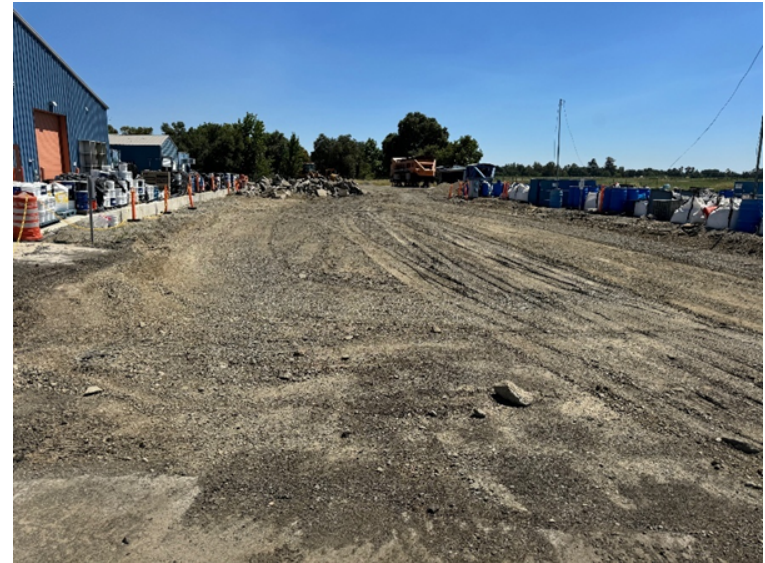
Figure 3.7: West Track after JPCP removal.
