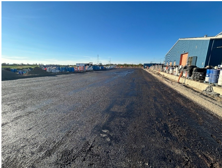
Figure 3.34: Prime coated aggregate base.
