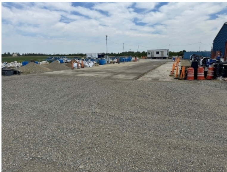
Figure 3.1: West Track prior to BMD construction.
