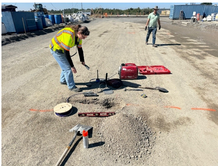
Figure 3.29: Pressure plate installation in the aggregate base.
