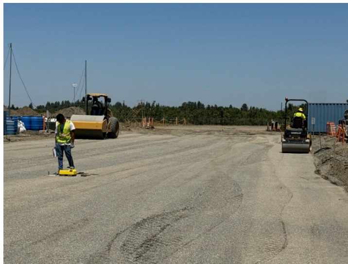
Figure 3.13: Aggregate base testing with nuclear gauge.
