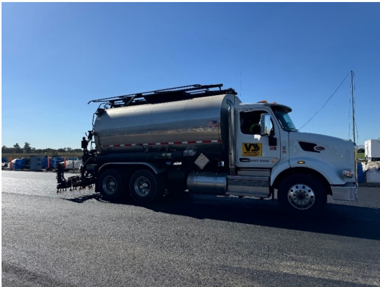
Figure 5.6: Tack coat application by truck sprayer.
