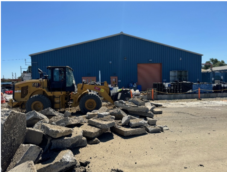
Figure 3.4: Loader removing concrete pavement.
