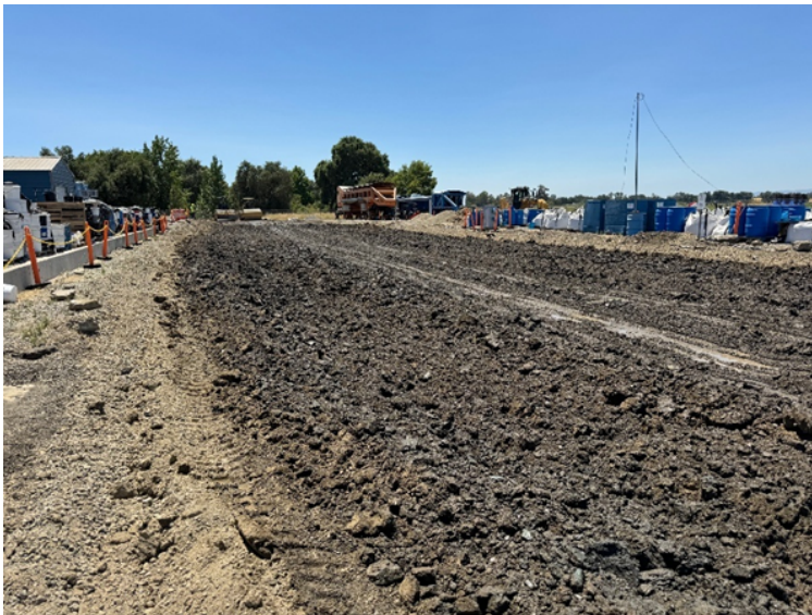
Figure 3.8: Ripping subgrade.
