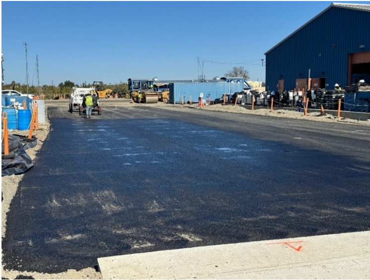
Figure 5.5: Tack coat application by hand sprayer.
