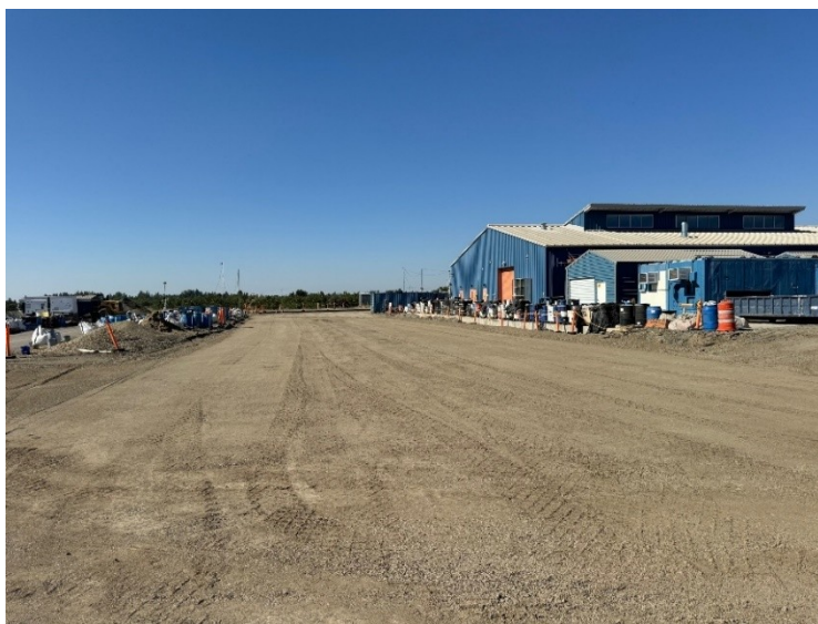
Figure 3.12: Graded and compacted Class II aggregate base.
