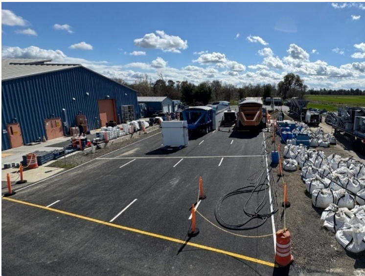
Figure 5.14: HVSSs on Lane 1 and Lane 3 rutting evaluation sections.
