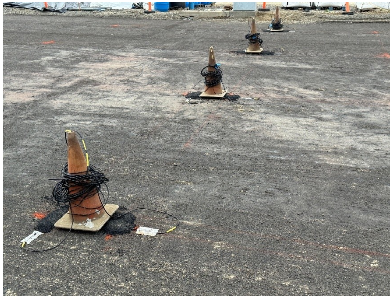
Figure 3.30: Strain gauges on the surface of the aggregate base.
