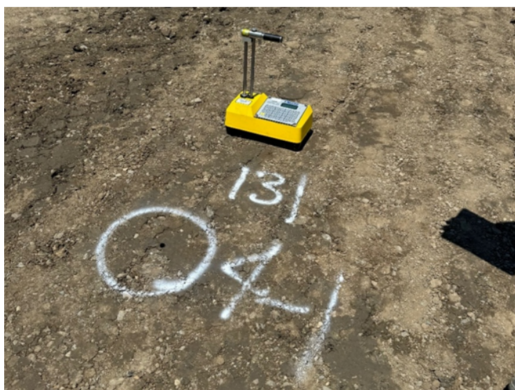
Figure 3.10: Nuclear gauge evaluation of subgrade soil.
