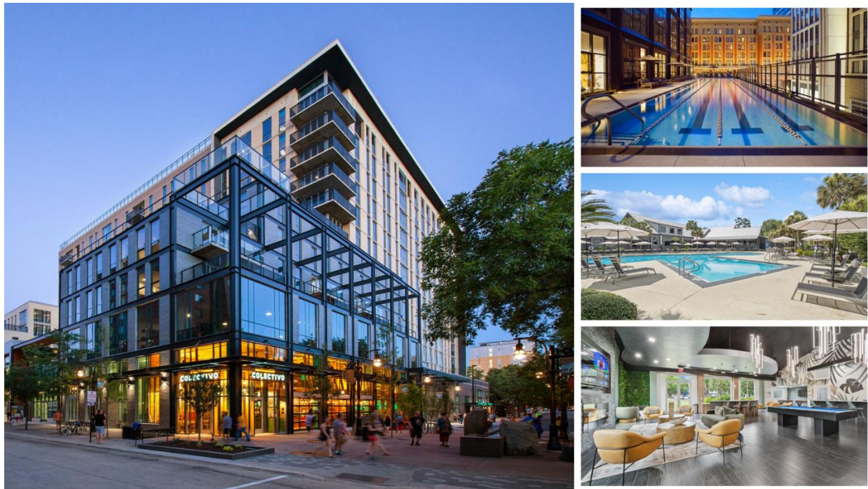
Photo Credit: Greystar Worldwide LLC & FPA Multifamily LLC
