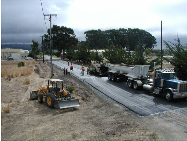
Figure 2.13: Asphalt concrete placement
