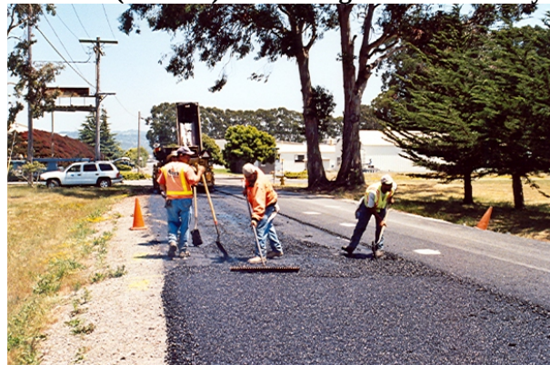
Figure 5.3: Overlay placement (MB4-G).
