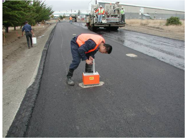
Figure 2.14: Nuclear density testing
