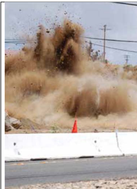
Figure 18. Bedrock blasting for SR-76 Middle (2010)
