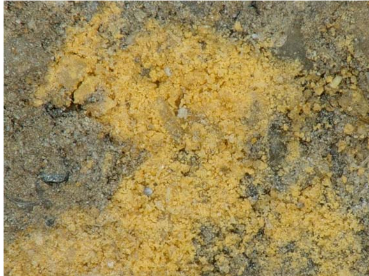
Figure 28: Powdering
