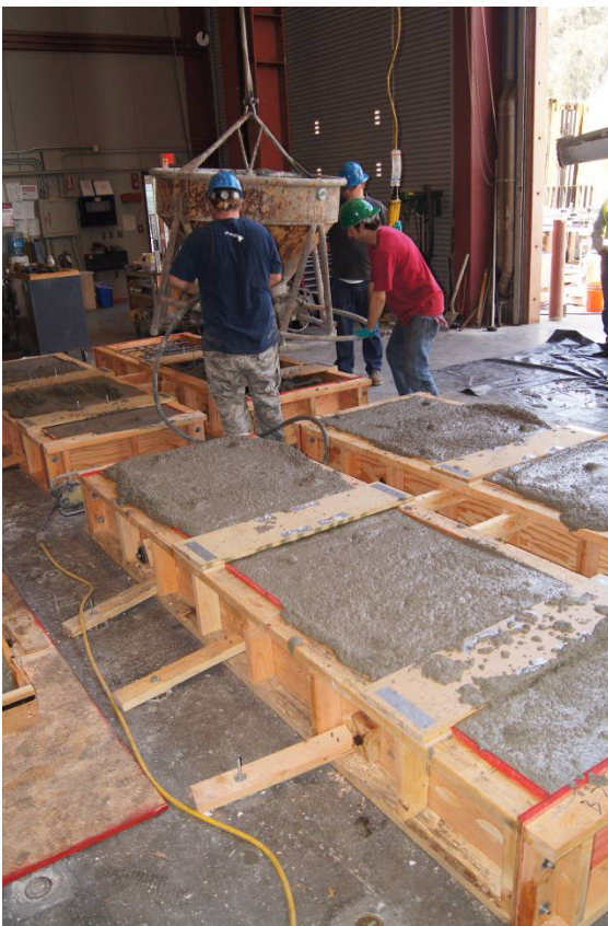
(a) Foundation form filling
