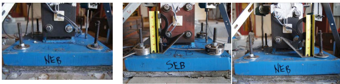
Figure 5-74: Configuration 3 - Typical condition of baseplate connections following Service, Design, and Maximum motions (from left to right)
