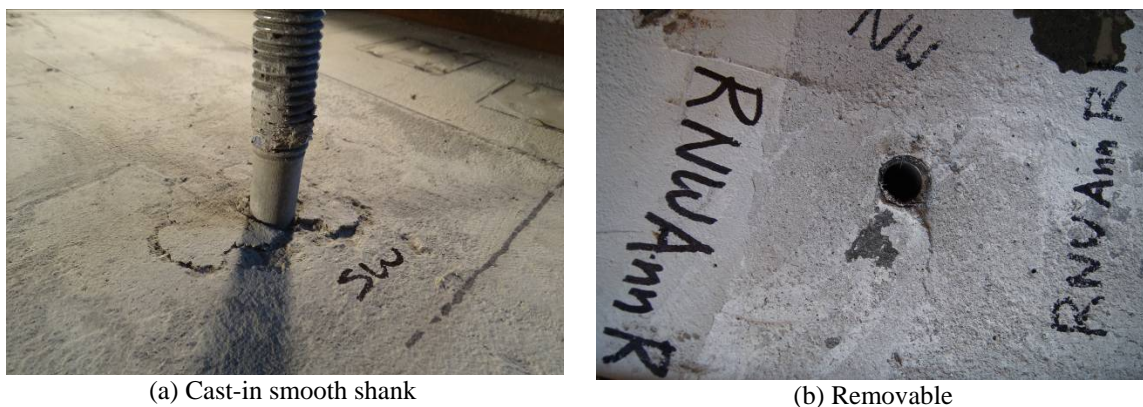
Figure 3-35: Post-test condition of concrete surface – shank condition comparison
