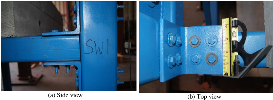
Figure 5-46: Configuration 1 - condition of beam-column connections at end of strong motion sequence
