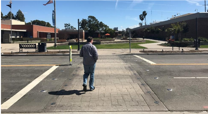
Figure 5.4. Blinking lights and different paving material in downtown El Segundo calm traffic provide and provide pedestrian safety. Source. Author
