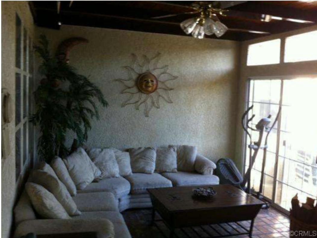
Figure 5.3. An unpermitted rear addition in Bellflower. Created by enclosing a formerly open air rear patio, it appears to exhibit a relatively high level of construction quality. Photo from www.redfin.com .
