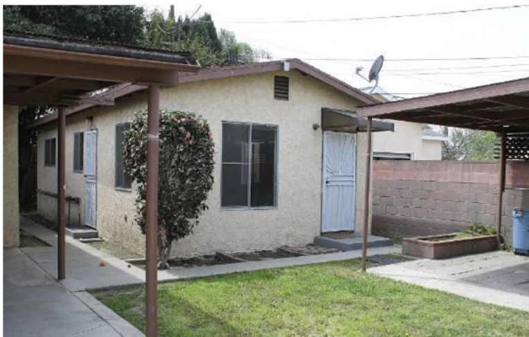
Figure 5.7. An unpermitted back house on a residential property in Lynwood. Source: www.redfin.com .
