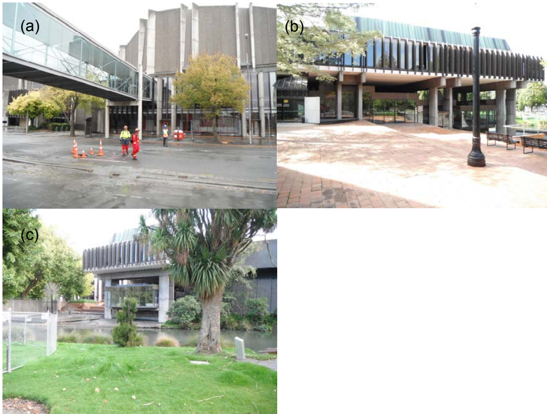
Figure 4.9.2. Photos of the (a) auditorium as viewed from the north, (b) the restaurant as viewed from the west, and (c) restaurant as viewed from Victoria Square Park to the south, Photos were taken March 2011.
