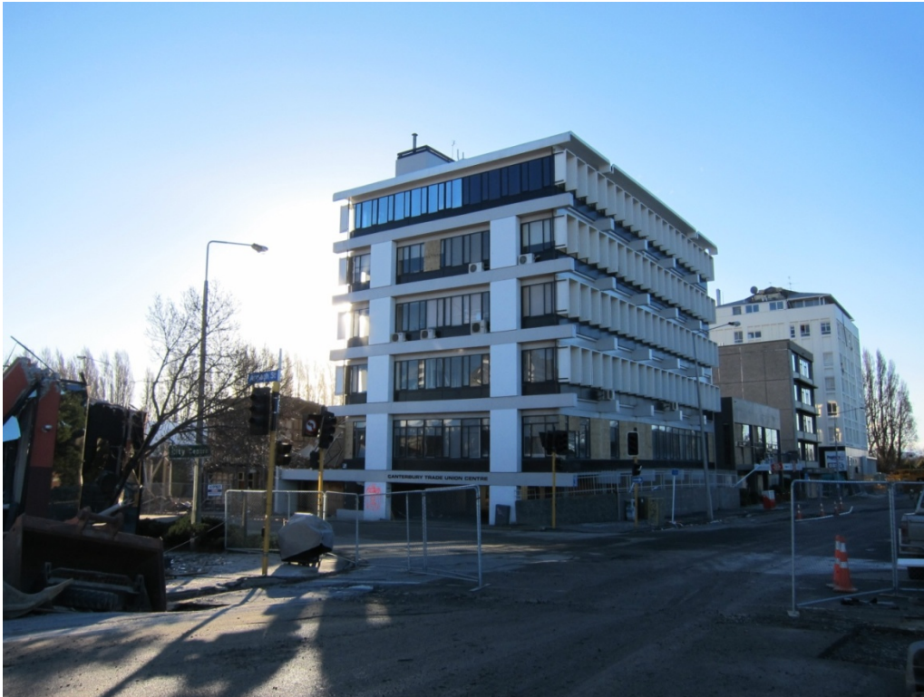
Figure 4.3.2. Photo of the CTUC building taken in July 2011, following several damaging earthquake events (photo courtesy of M. Taylor).
