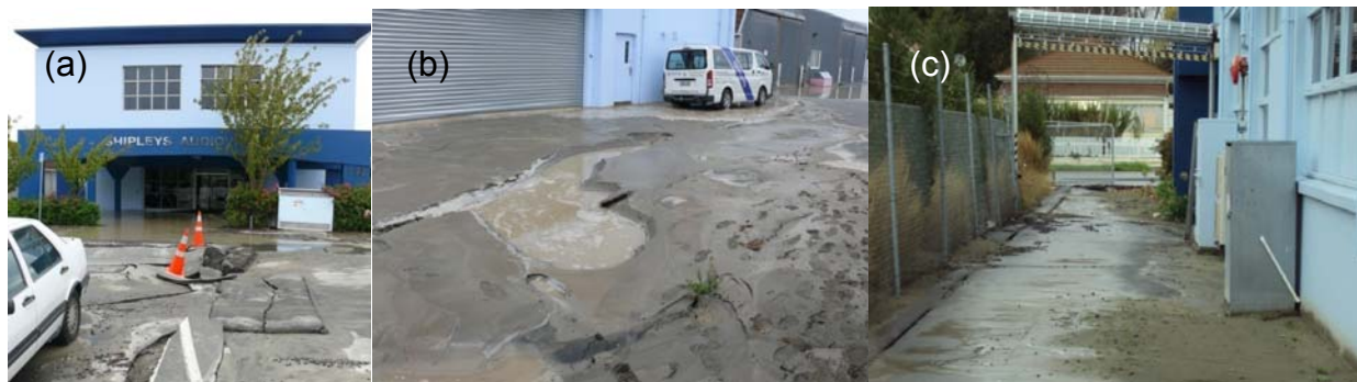
Figure 4.4.4. (a) Views of the south end and (b) north end of SA building taken approximately 2 hours after the Christchurch earthquake. (c) Photo of the east side of the building taken June 5th, 2011. (Photos courtesy of Shipleys Audiovisual Ltd.)
