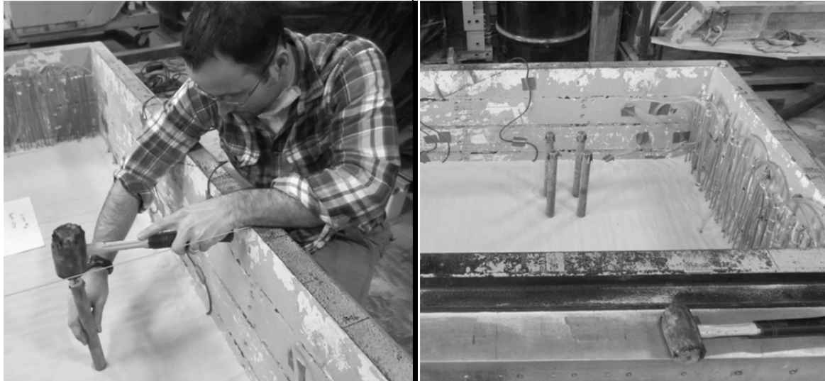
Figure 3.2.14. Installation of model piles.
