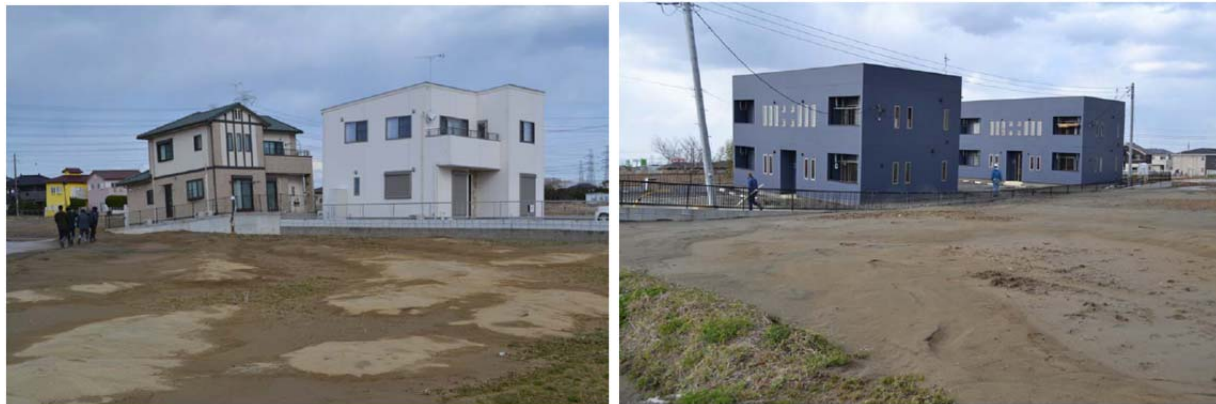
Figure 2.2.3. Settlement and tilting of residences in Kamisu City (N35.917, E140.642). Photographs from GEER Association Report No. GEER-025a (Ashford et al., 2011).
