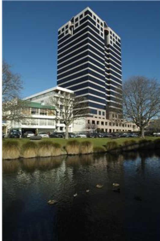
Figure 4.6.1. Photo of the PWC Building Prior to the Canterbury Earthquake Sequence (from Colliers International New Zealand Ltd., 2009)
