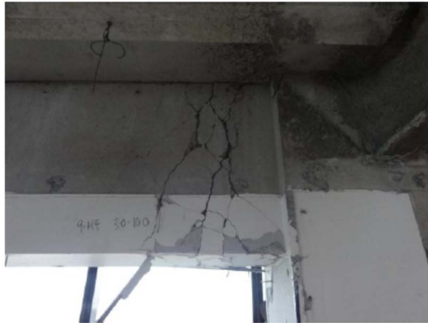
Figure 4.6.15. Photograph of beam plastic hinge (from Pampanin, 2012).
