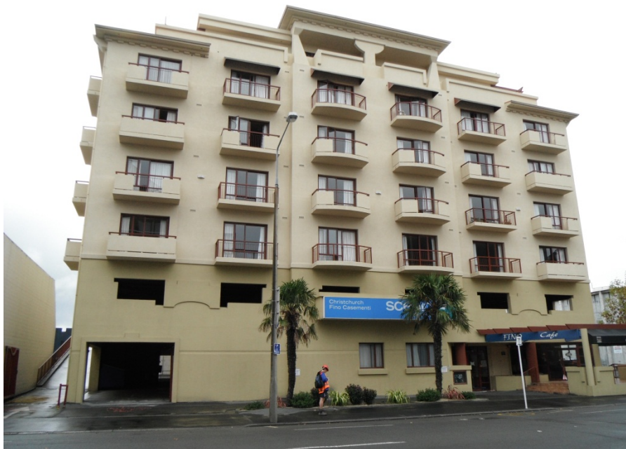
Figure 4.8.1. Photo of the SCH Building from March 2011.
