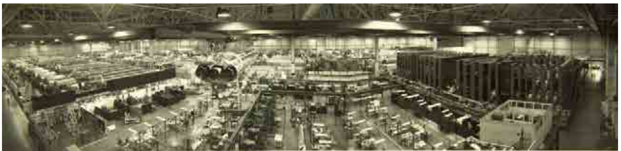
3.7. Convair Division, General Dynamics Corporation, Kearny Mesa Plant and Personnel , ca. 1955–1969. SDASM Archives, no. 10_0006256.
