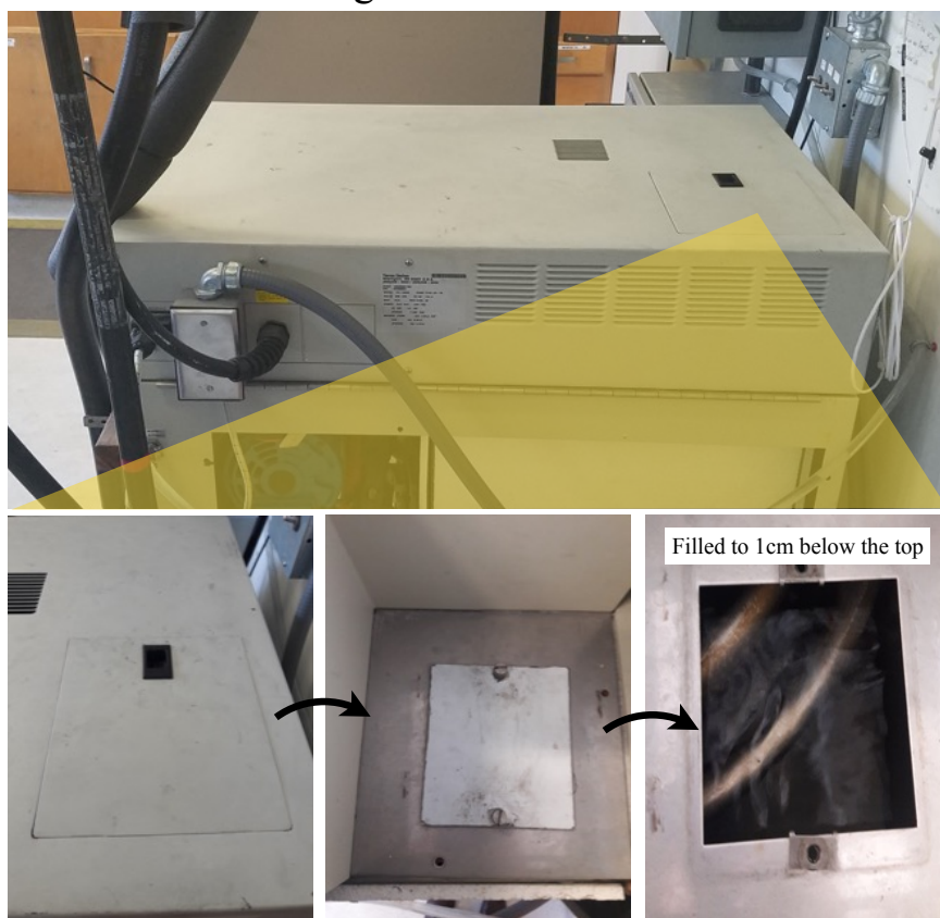
Figure 7.18: The lab chiller is filled by removing the two panels at the top of the lab chiller.
