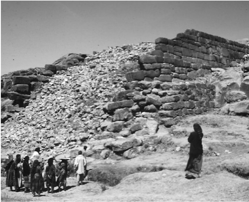
Figure 3.9. Sedd al-Ajmar severed by high-energy floods. Photo by T. J. Wilkinson.
