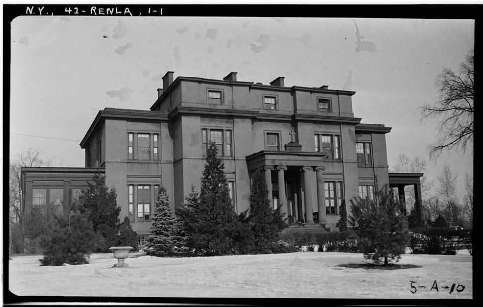
Fig. 92 Frederic Diaper, Beverwyck Manor as St. Anthony-on-Hudson Seminary, c. 1839. Rensselaer, NY. Photo from Historic American Buildings Survey, 1936.
