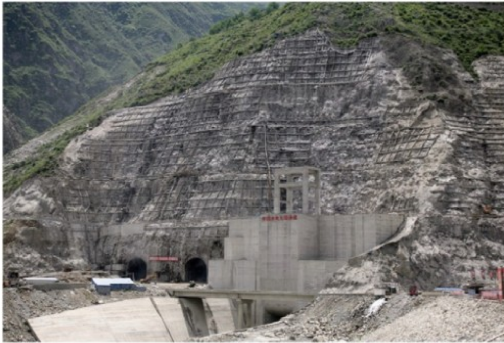
Fig. 21. Overall view of the HJP intake slope after completion.
