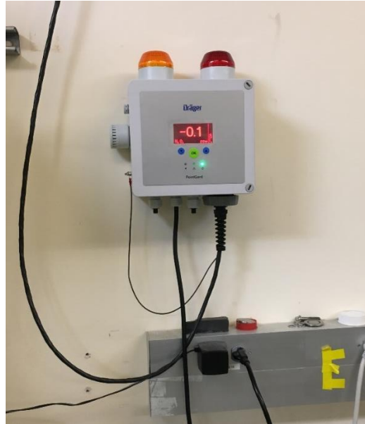
Figure D.5 Hydrogen peroxide monitor located on south wall of Eng V 1021.
