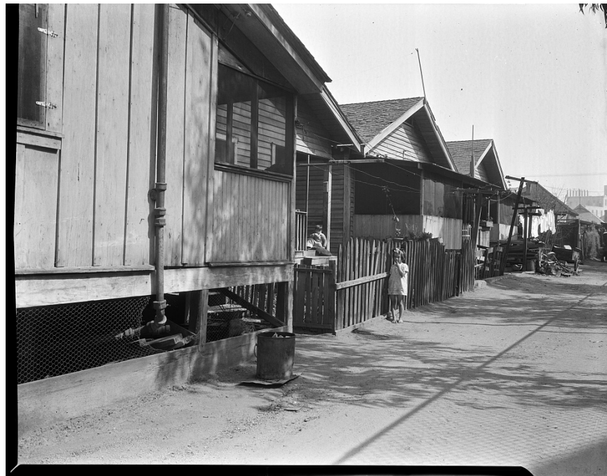
Figure 23: "Mexican quarter" of Los Angeles, to be torn down to make space for the new Union Railroad Station, 1936, Dorothea Lange, photographer. FSA - Office of War Information Photograph Collection, Library of Congress.
