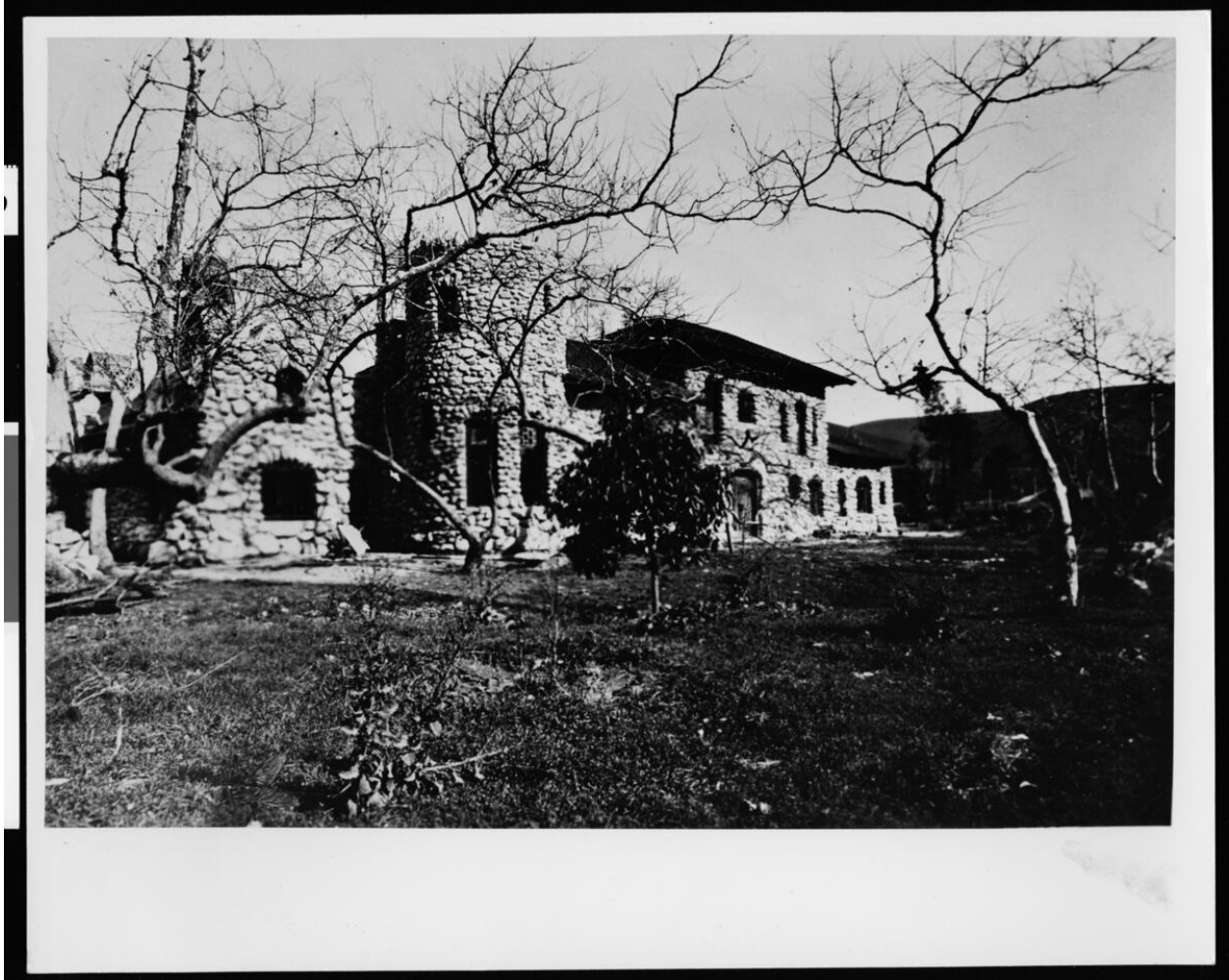
Figure 9: Exterior photo of Lummis' house, "El Alisal," ca. 1898-1910, featuring arched openings and a cylindrical rock tower (CHS, USC, DC)
