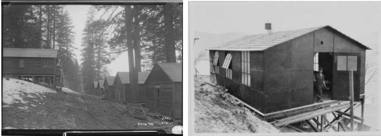
Figure 21: Bunkhouses for workers at Big Creek, including prefabricated, portable redwood bunkhouses made by Pacific Readycut Homes, 1920 (left) and metal “portab” bunkhouses for 10 men, 1922 (right), SCEPN, HDL
