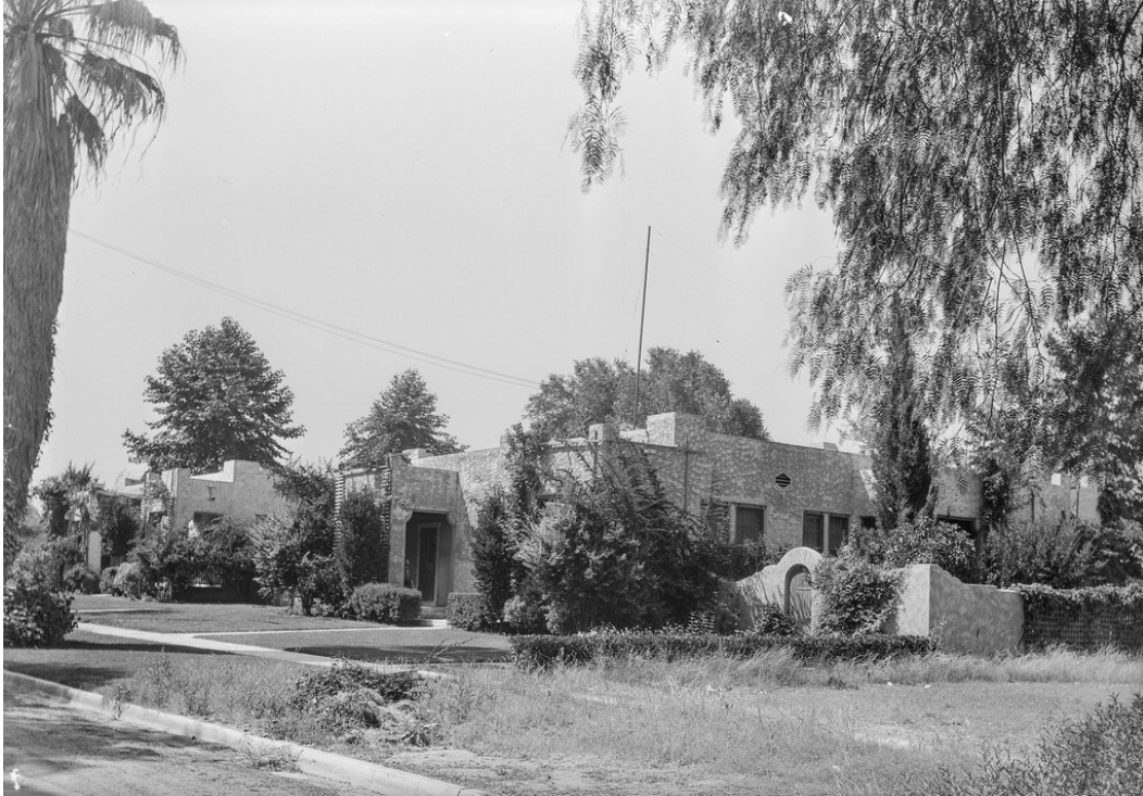
Figure 20: Employee housing on Jackson Avenue, cs. 1930-1950, Box 146, SIM
