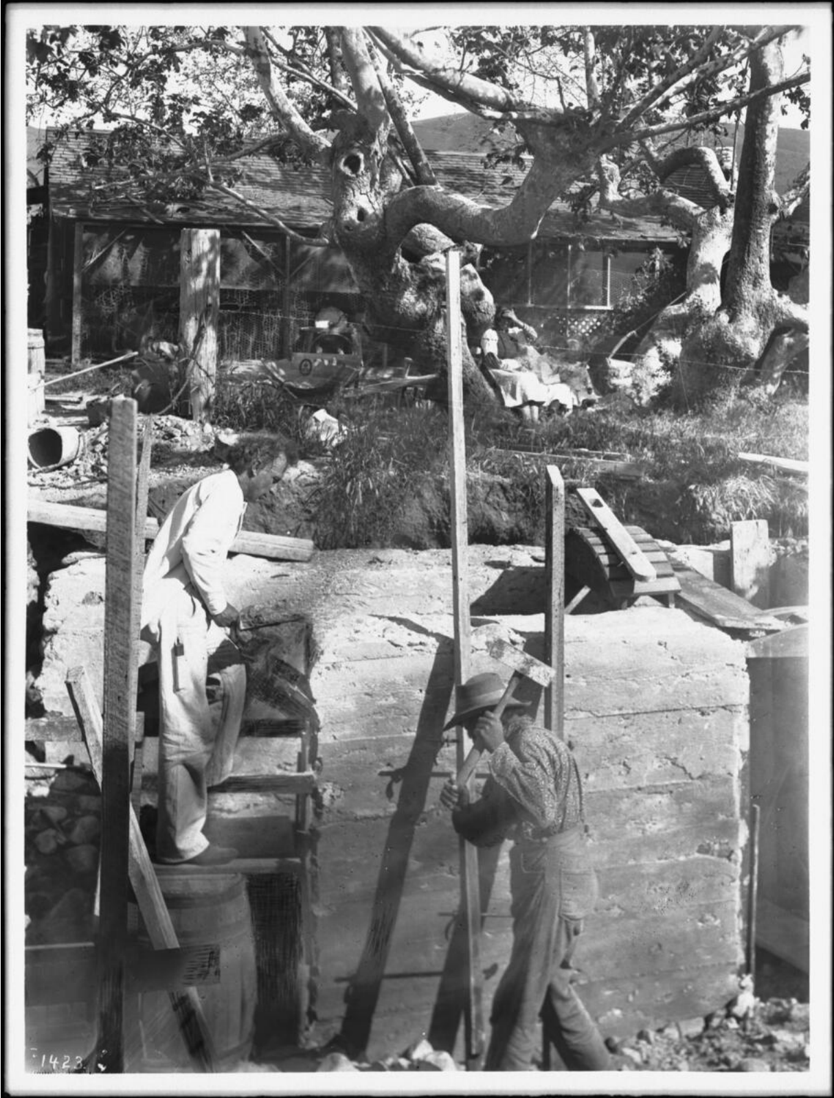
Figure 10: Lummis with construction worker (likely Isleta Puebloan), excavating for the construction of his home, El Alisal (CHS, USC, DC).
