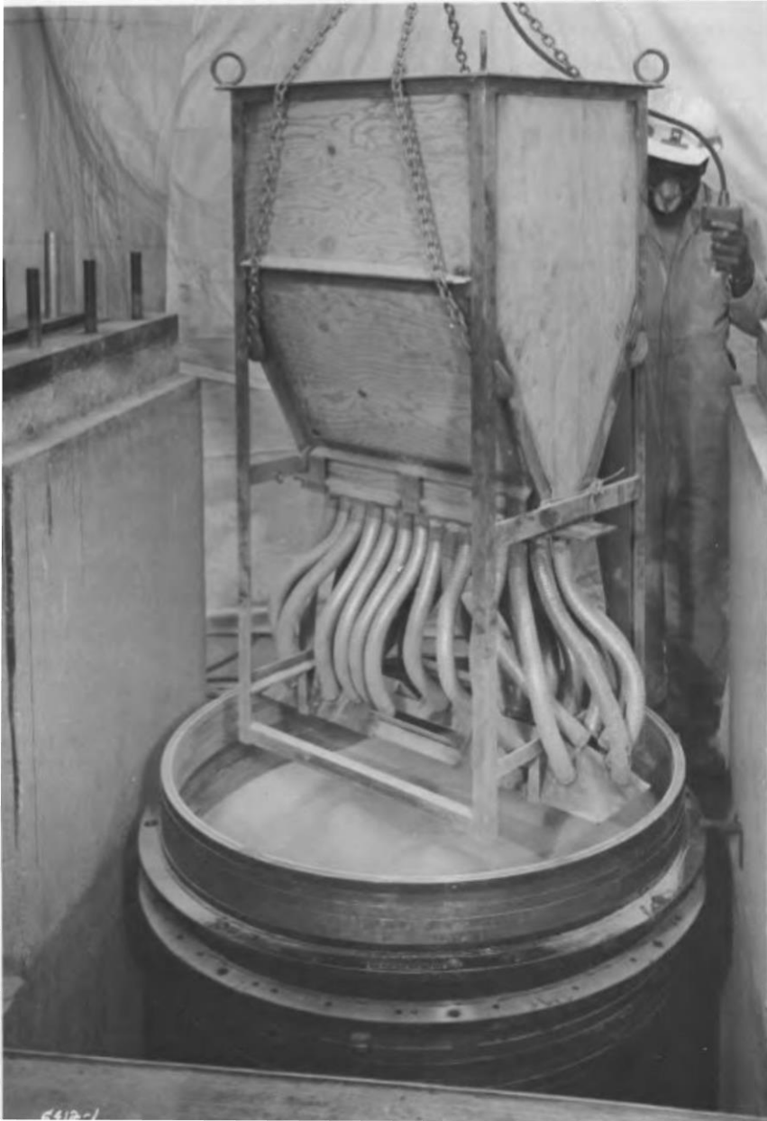
Figure A-5: Rotating Rainer Used in WES Study (from Biegansky et al., 1976)
