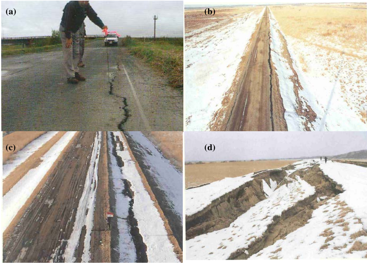
Figure 2.5 Photographs after the 1993 and 2003 earthquakes showing the various damage levels. (a) Level 1, with minor cracking and no subsidence, (b) Level 2, with 20-30 cm of subsidence and cracks on the exterior face (c) Level 3, with subsidence of over 30 cm and (d) Level 4, with 60-225 cm of subsidence and 6 m wide cracks (KDCO 1994, 2004).
