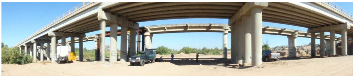
Figure 1. October 2013 site investigation underway at the San Felipe Bridges. Highway bridge is in the foreground; railroad bridge in background. Colorado River, obscured by vegetation, flows under bridges on left side of photo.
