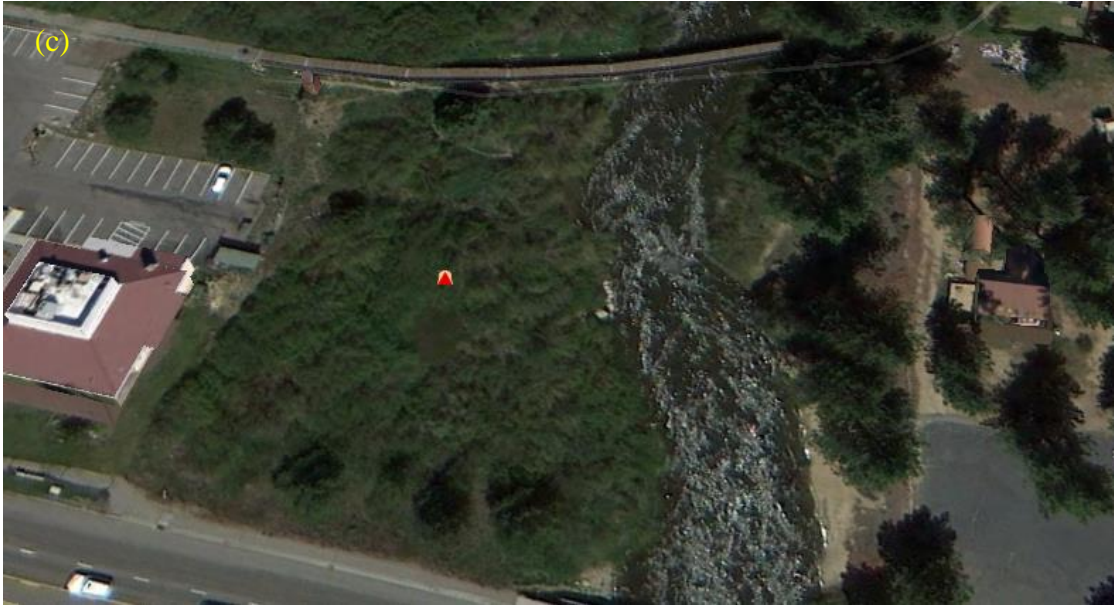
Figure A.1. (a) Q_s vs Q relationship from 1971 to 1992, (b) Q vs Gauge Height, and (c) photo image of site location from Google Earth at Upper Truckee River at South Lake Tahoe, CA.
