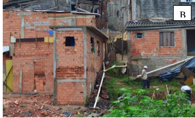
Figure 2.1. 1A and 1B. Fig. 2.1A illustrates a mixed-material building in a favela in São Paulo city (Source: Goto, 2012). Fig. 2.1B illustrates brick buildings in one of São Paulo's favelas. Both brick and mixed-material buildings are precarious, but mixed-material ones are less resistant than brick buildings and can be easily destroyed (Source: Goto, 2012)
