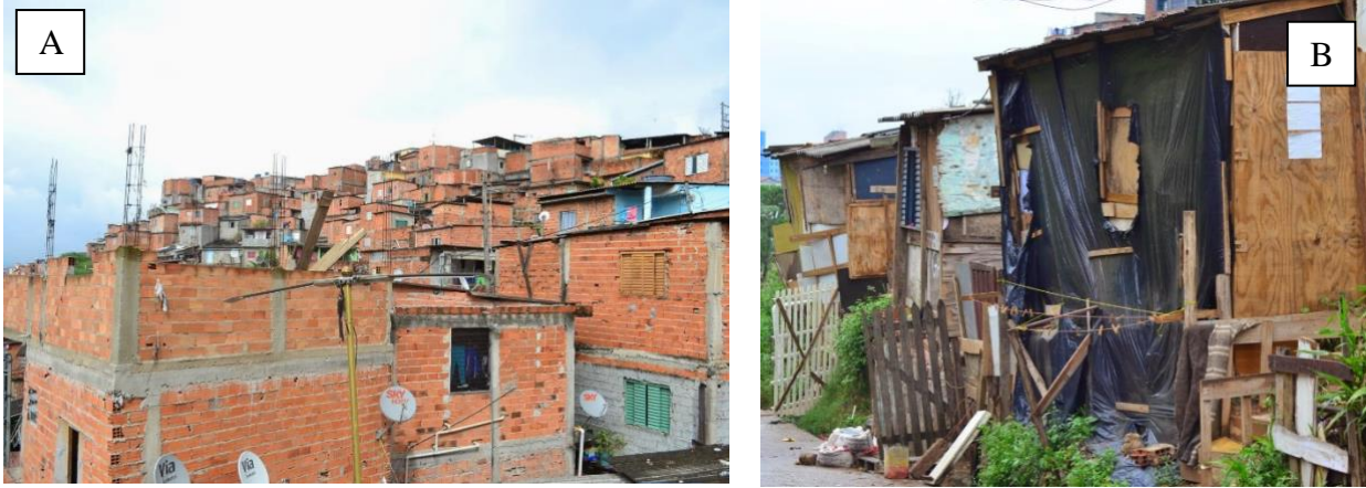
Figure 3.5. 3.5A and 3.5B. Fig. 3.5A. Brick dwellings are the ones with most of the dwellings made with bricks. They are more resistant than wood and mixed material dwellings. Fig. 3.5B . Mixed material dwellings combine different materials and the dwellings are very precarious
