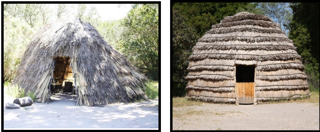
Figure 36 Structures that represent Native housing at Mission La Purisima. Source: Author's personal collection.
