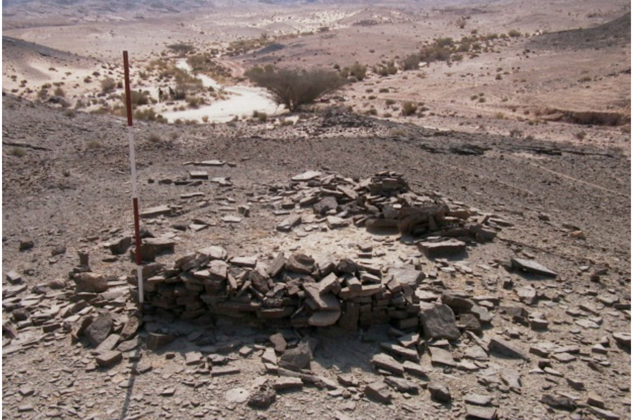
Figure 4.32: Poorly preserved standing architecture of Building 5305 in 2002. (Photo: courtesy UC San Diego LCAL.)
