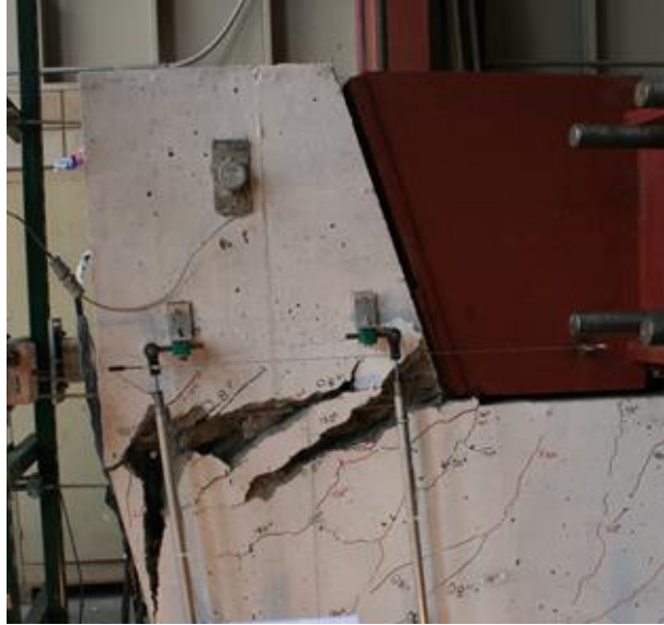
Figure 6.62 Deformed configuration of shear key 9A at the end of the test
