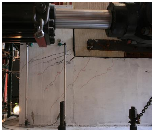
Figure 6.102 Cracks on the east face of shear key 10B at 250 kips
