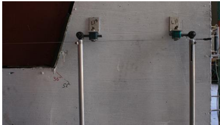
Figure 6.85 First diagonal crack observed on the east face of shear key 10A
