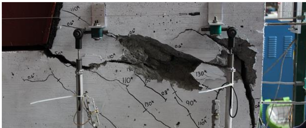
Figure 6.34 Sliding shear plane from the east face of shear key 8A
