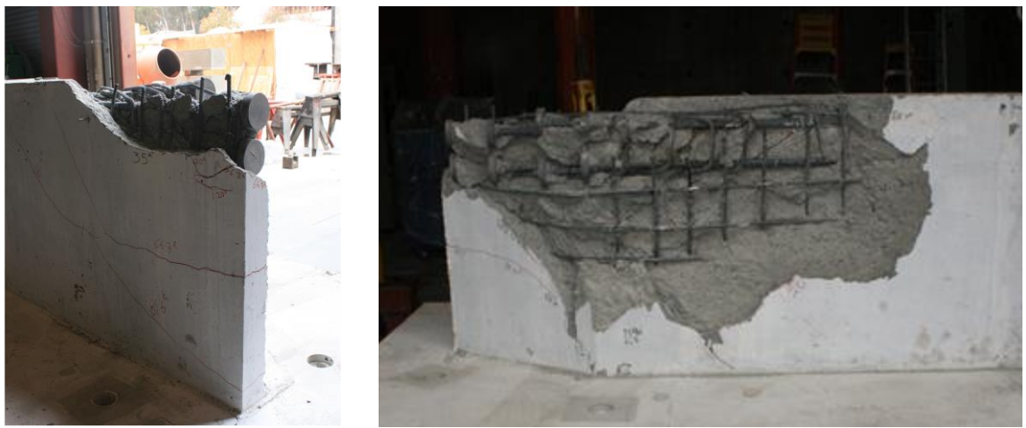
Figure 8.34 Shear plane from the southeast side (left) and from the northwest side (right) after removing shear key 12B
