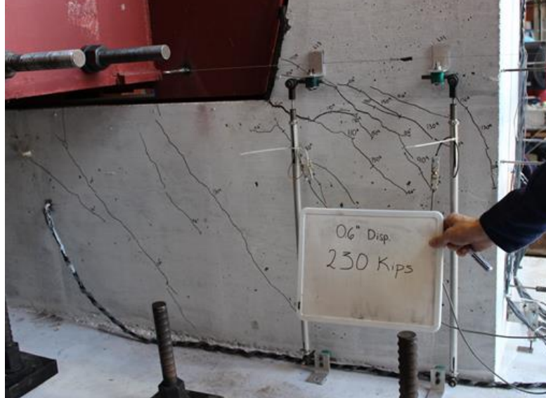
Figure 6.33 Cracks on the east face of shear key 8A at 230 kips load
