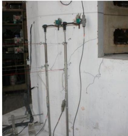
Figure 8.17 First cracks observed on the northwest side of shear key 12A
