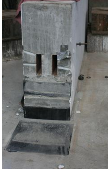
Figure 7.26 Stem wall and neoprene pads after shear key block was removed in Test 4
