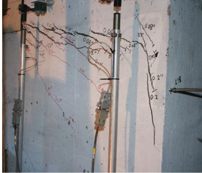
Figure 6.47 Sliding plane from the west face of shear key 8B
