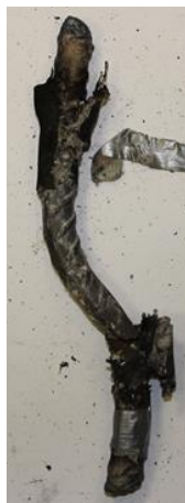
Figure 5.40 Angle of kink observed in vertical reinforcement of shear key 7B
