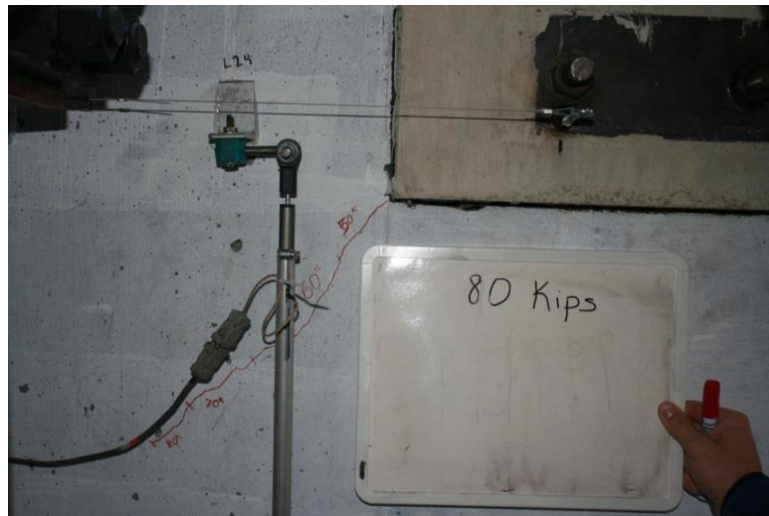
Figure 6.45 Propagation of first diagonal crack on the east face of shear key 8B
