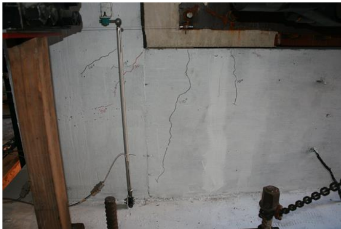
Figure 6.72 Propagation of first diagonal crack and additional cracks on the east face of shear key 9B
