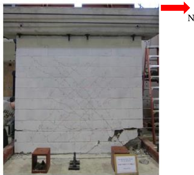
Figure 4.24 Damage at the end of the test of Ahmadi (2012)
