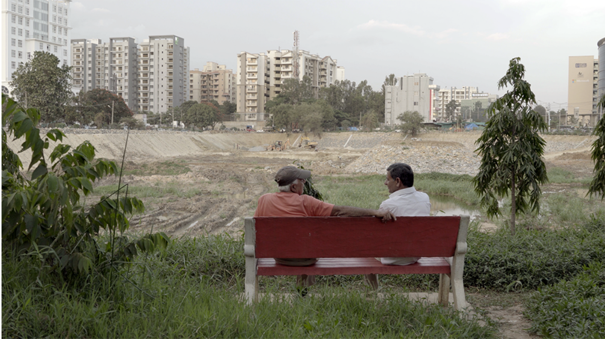
Figure 11: view of Iblur lake under construction
