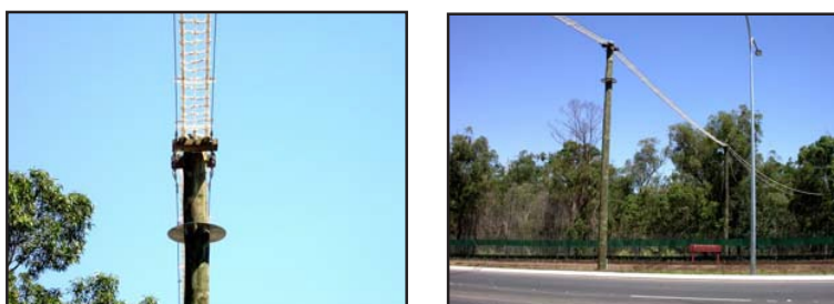
Figure 11. 60m-long rope ladder-style arboreal overpass erected in open forest habitat in Brisbane, Queensland. (Photos by Pauline Fitzgibbon)
