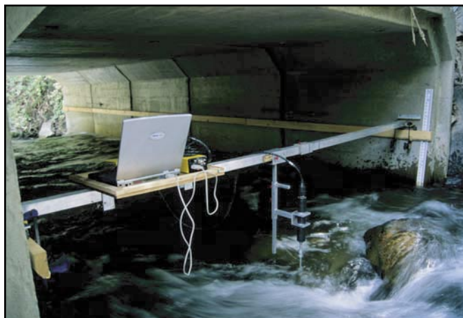
Figure 3A. ADV harness in culvert 2 inlet region.
