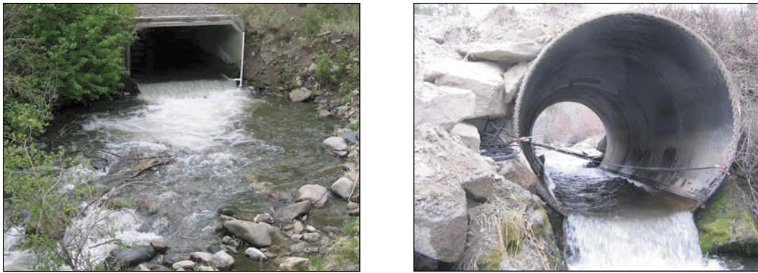
Figure 2A. The outlet of culvert 1, a box pipe (l), and the outlet of culvert 4 (r).
