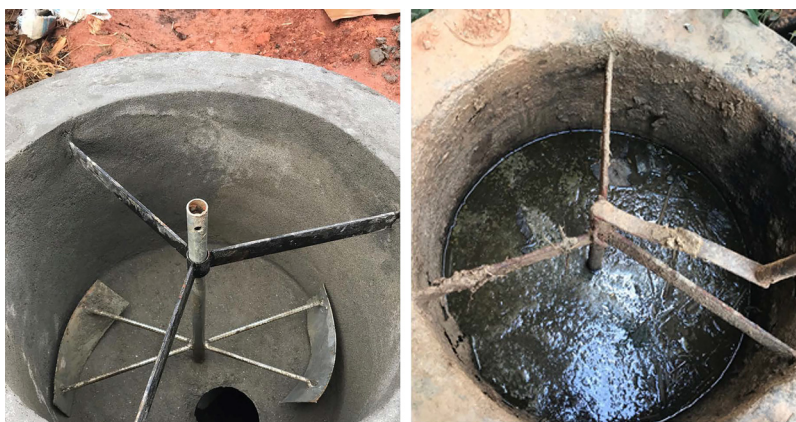
Figure 1. Animal dung is collected, combined with water and urine, and mixed into biodigesters via an inlet with an agitator, shown here after construction (left) and after being used (right).
