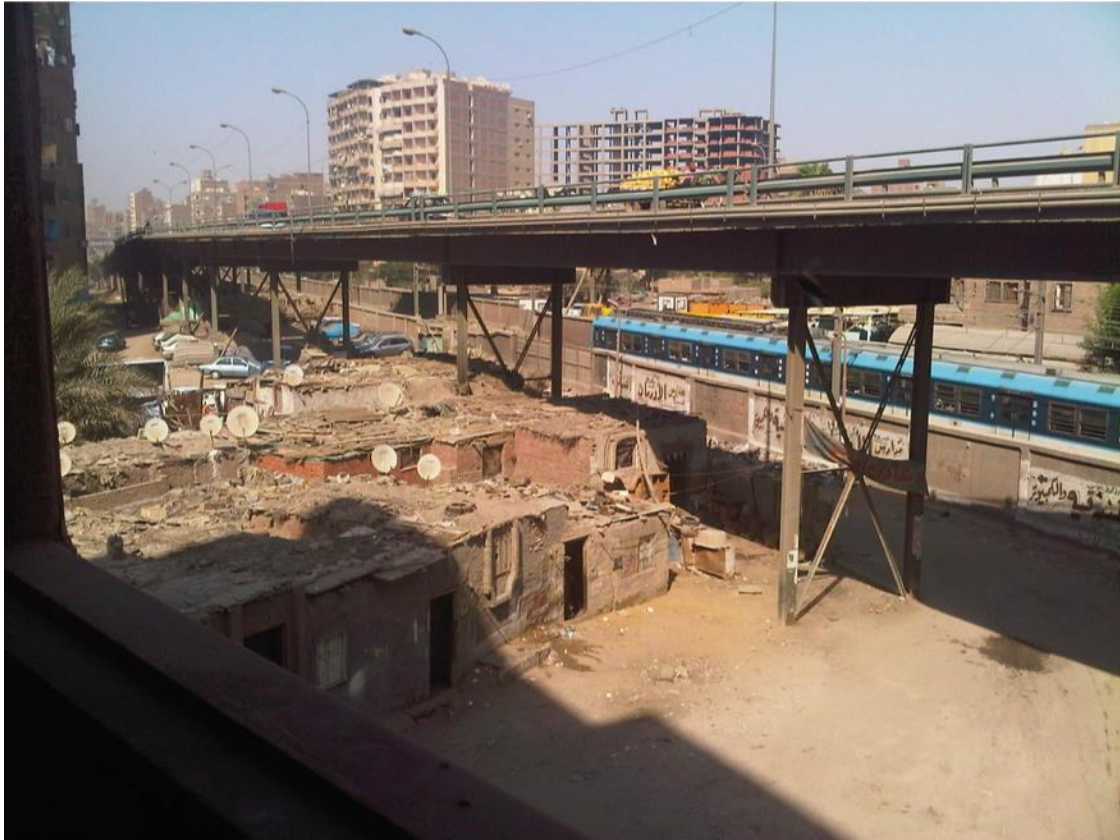
Figure 4. View of shanty town built illegally over a major gas line. View from Mosque with Cairo's commuter railway visible. Hizbt Nakhil. Photo by the author.
