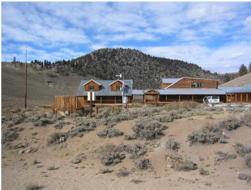
Figure 10. Crooked Creek Research Facility. Elevation 3094 m / 10,151 ft. View from south to north.
