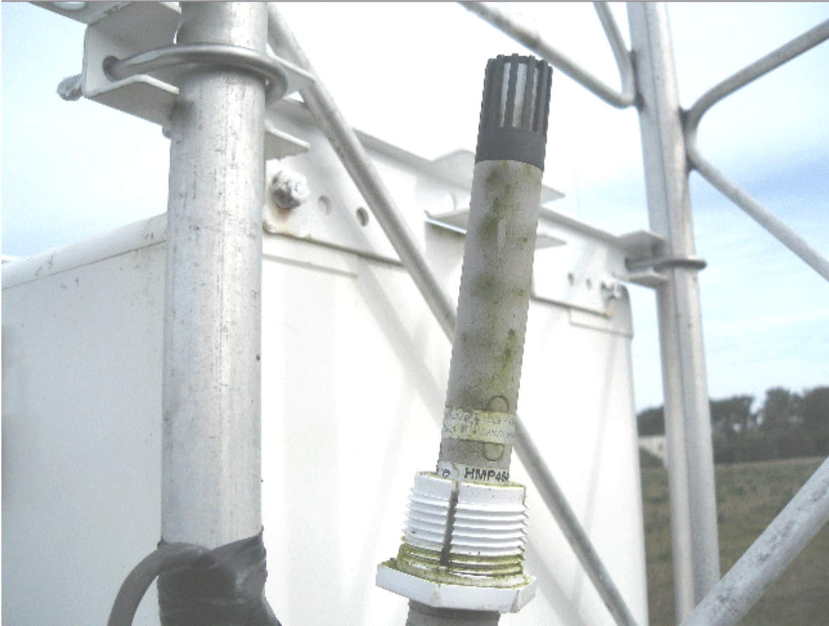
Figure 34. Point Reyes National Seashore RCA Building site. Radiation shield has been removed to reveal mildew and organic film covering portions of the support for the temperature and humidity sensors, which are located in the dark gray slotted area near the top of the photo.
