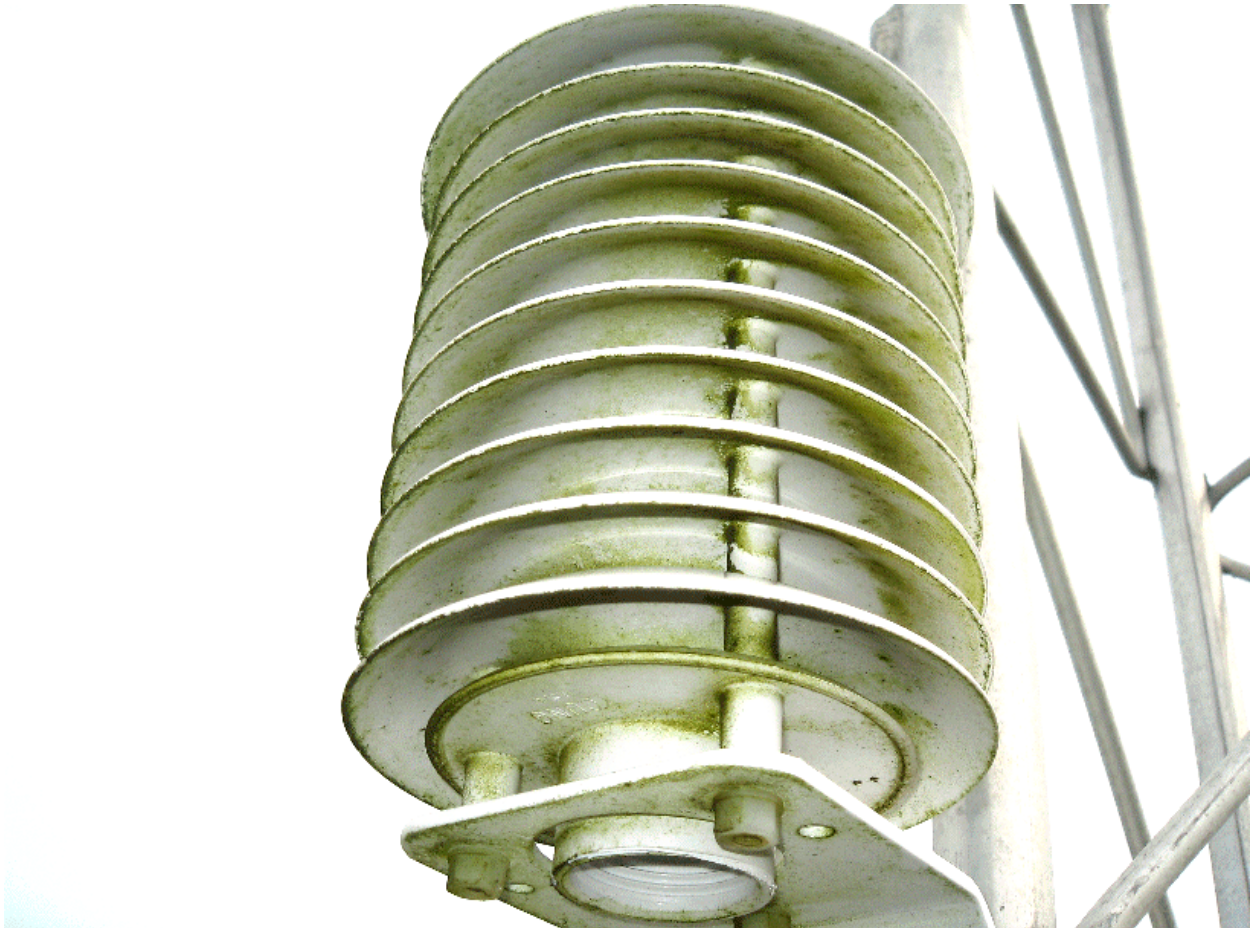
Figure 37. Thermometer shielding at Point Reyes RCA Building site, showing mildew and organic growth, 18 months after deployment. This causes extra heating on sunny days, and retains water for further growth. Material removed and cleaned.
