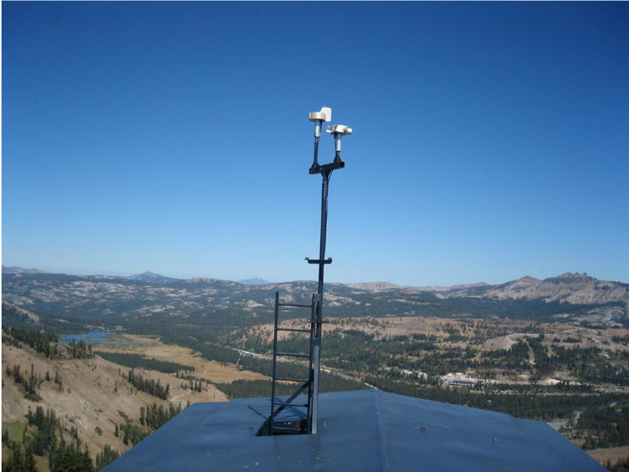
Figure 20. Taylor anemometer direction and speed sensors atop Mt. Lincoln (2539 m / 8330 ft). Mounted on top of summit building housing upper end of chair lift. Looking approximately toward northwest, with Castle Peak and Donner Summit to right, Central Sierra Snow Lab approximately behind left side of third rung of ladder from top.
