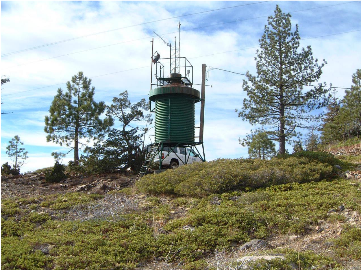
Figure 24. Photo of Cisco Butte climate station. Steel container formerly used to store equipment. Photo taken Nov 15, 2006 by Greg McCurdy.
