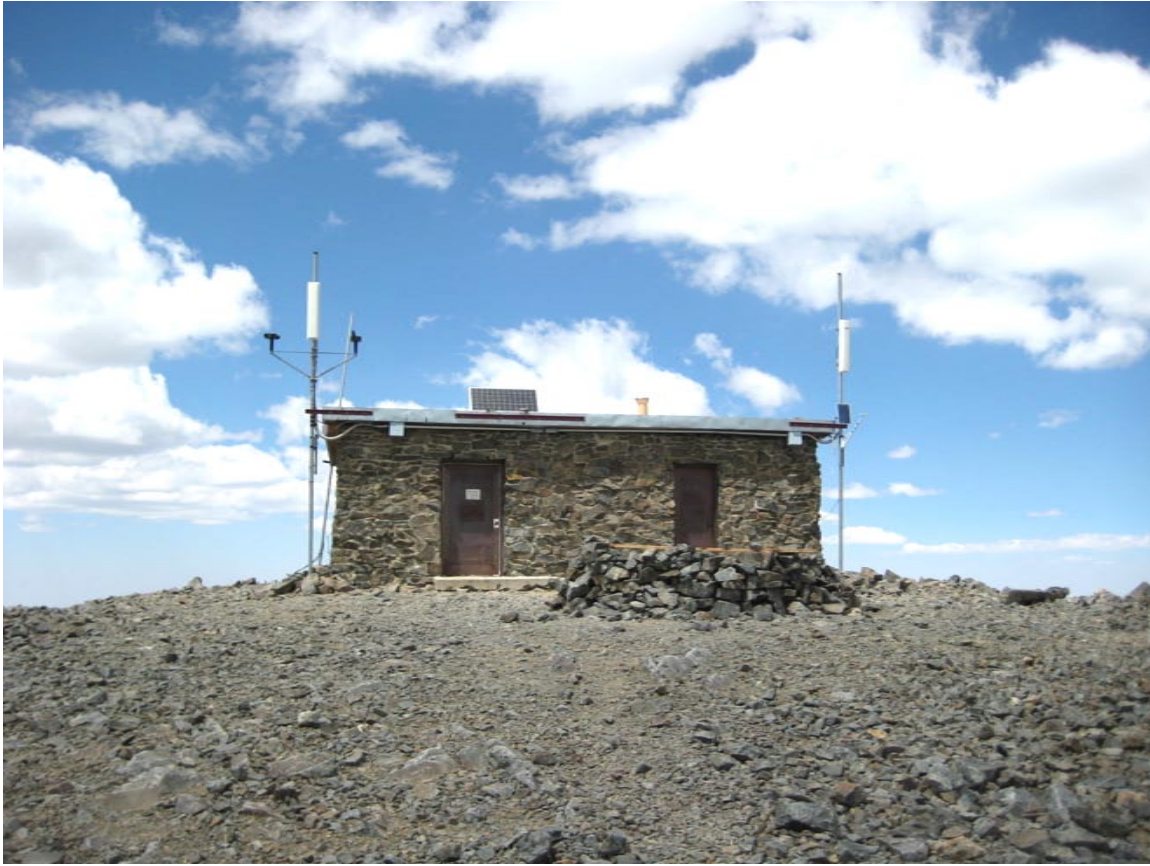
Figure 8. Long term monitoring equipment atop White Mountain Summit, 4342 m / 14246 ft. Anemometer and temperature/humidity sensors on left mast, solar radiation on right mast. All equipment is solidly bolted to the stone hut. Radio equipment extends above the mast. View from south to north.
