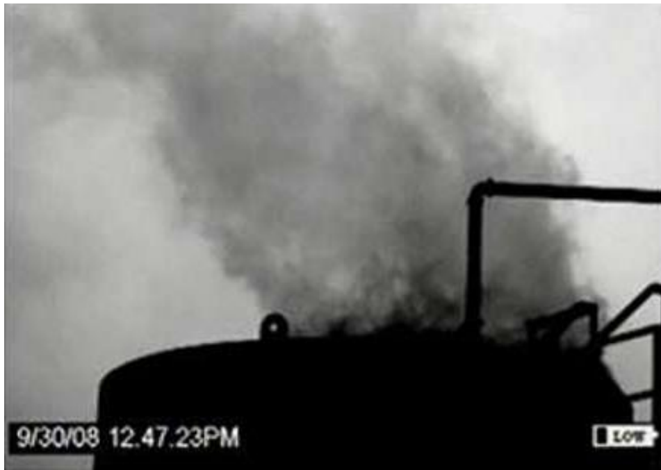
Figure 2.12. Methane emissions from the liquid storage tank (taken from [71])
