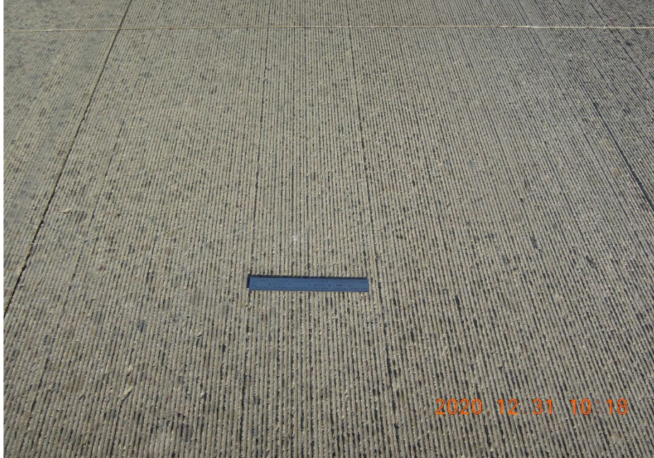
Figure 7.2: Grinded concrete surface.
