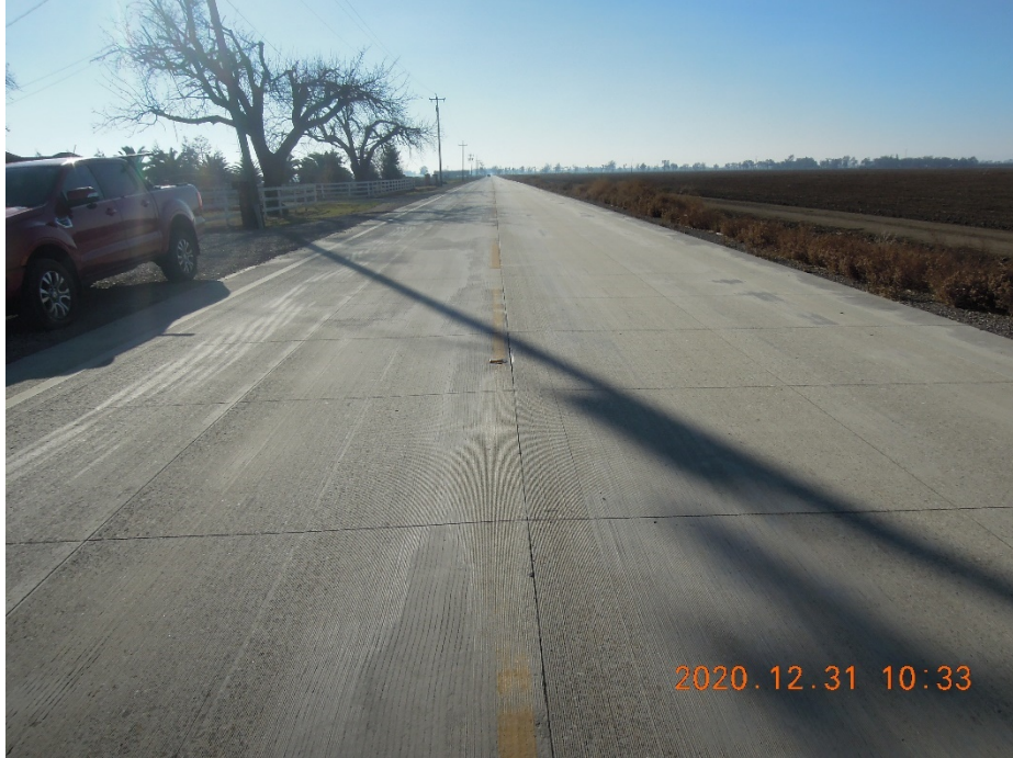
Figure 4.1: Typical appearance of the concrete overlay.
