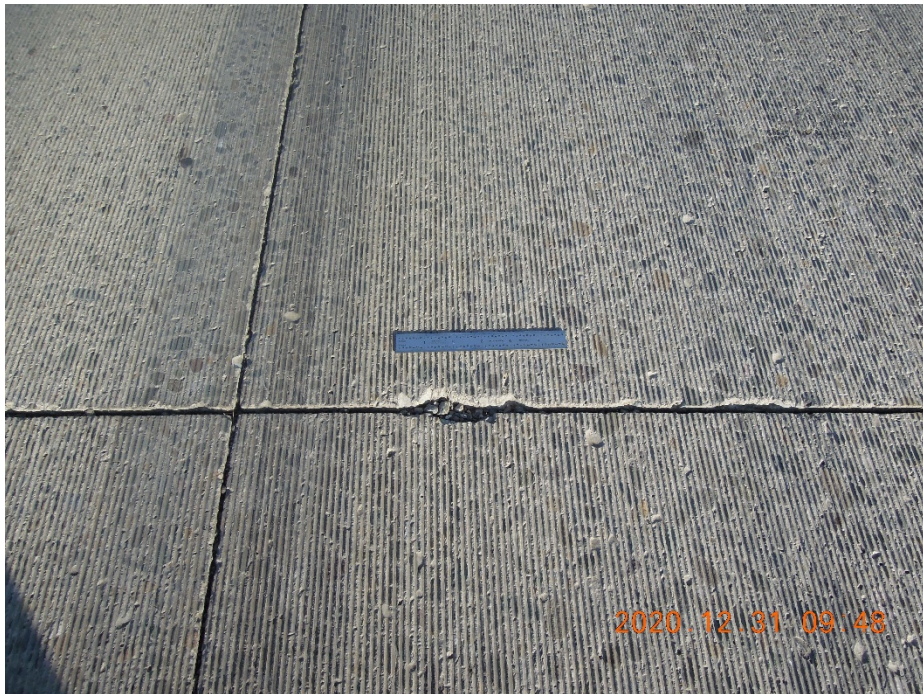
Figure 4.4: Low-severity spalling.
