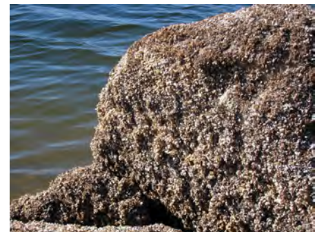
Figure 1-1. Mussel infestation exposed on rocks after a water draw-down. El Capitan Reservoir, San Diego County, CA. Photo Credit: Carolynn Culver
