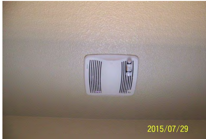
Figure 16 Data logger measuring temperature and relative humidity that was attached to a bathroom exhaust fan grille.
