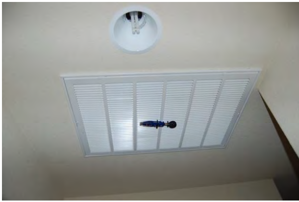
Power meter on the air handler (upper left photo), temperature/relative humidity sensor at the supply grill closest to the air handler (upper right photo), digital anemometer at the return grill (lower photo)
