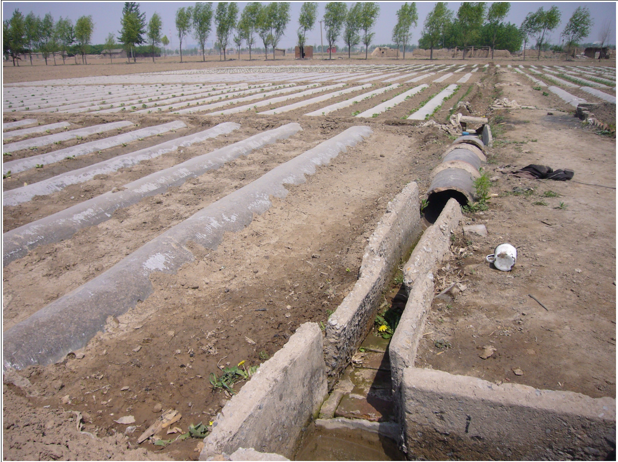
Makeshift irrigation ditch built by one farmer to carry water from his house to the fields.
