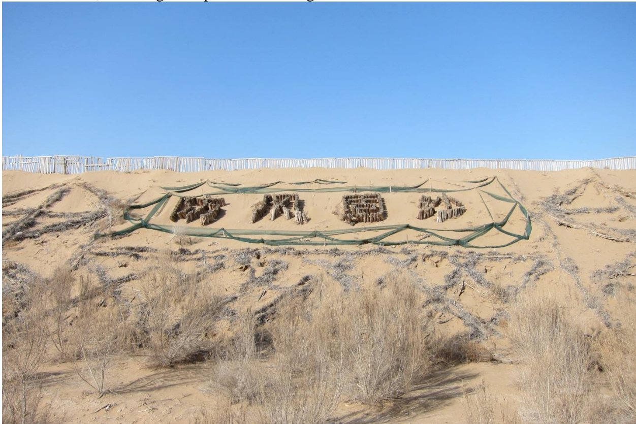
Figure 7: Laohukou, 'Mouth of the Tiger' Three Norths Shelterbelt demonstration site. Straw checkerboard barriers are laid out in an uncharacteristically aesthetic pattern, underscoring the spectacular nature of this demonstration zone. A slogan has been written on the dune in sticks and surrounded decoratively by nylon barriers. The slogan reads "Block the Wind, Hold the Sand"
