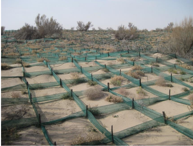
Figure 6: at a desertification engineering demonstration zone, a grid of nylon netting acts as a sand barrier to catch sands in their movement and to block winds at the surface. These nets aim to neutralize the effects of wind and create a tiny stabilized square where pioneer species can establish.
