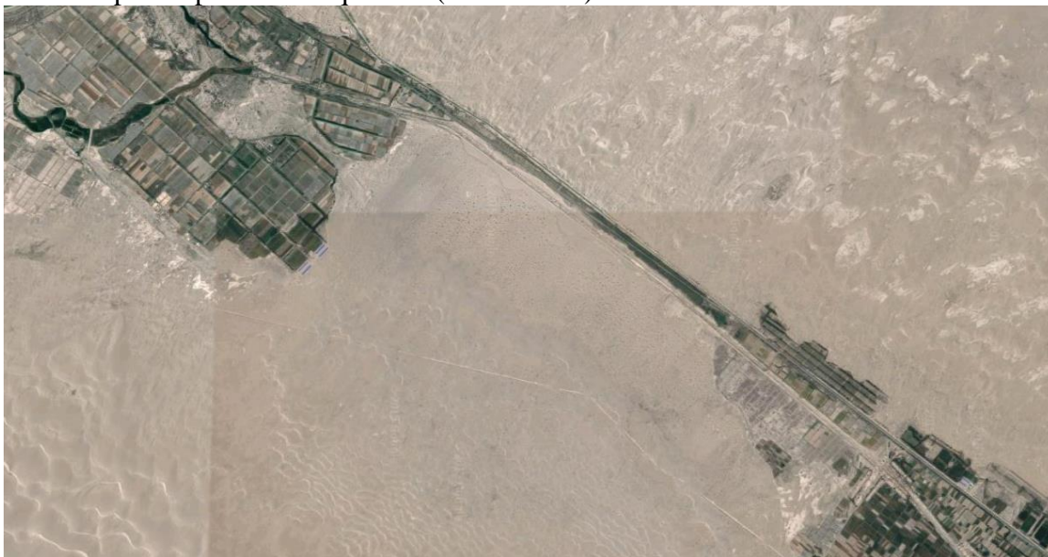
Figure 13: Minqin County’s single road and aqueduct, with desert on either side.
