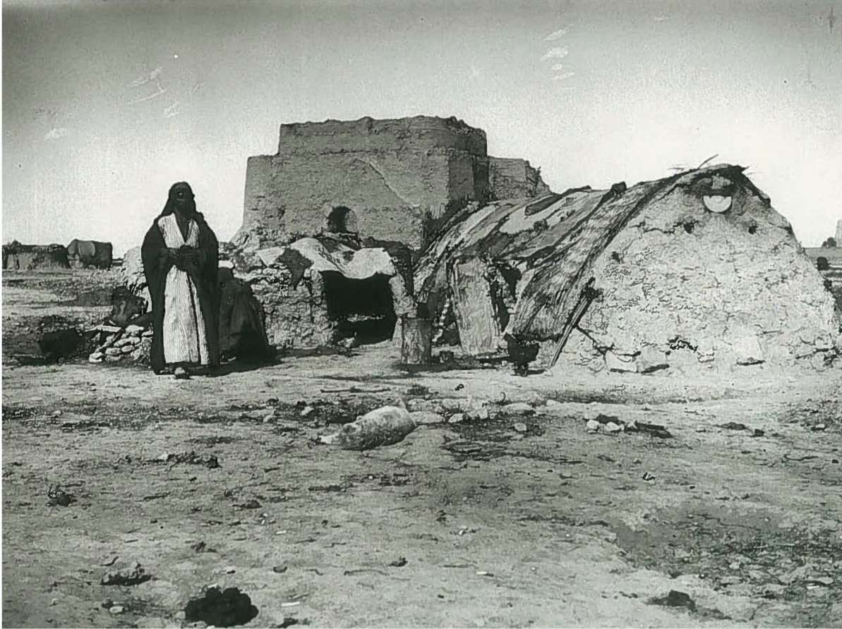
Fig. 2.4 Kamil Chadirji, "Typical sarifa (mud and reed hut) of the 1930s and its dweller, outskirts of Baghdad, 1931," from The Photography of Kamal Chadirji
