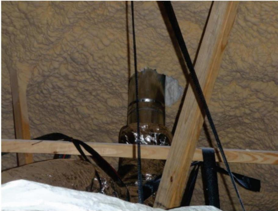
Figure 8 Example picture of gaps surrounding roof vent pipe penetrations. Source: Prah and Shaffer (2014).
