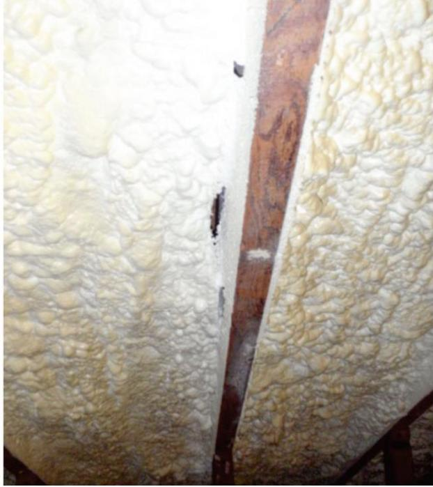
Figure 7 Example image of closed cell SPF delamination from roof framing member. Source: Prah and Shaffer (2014).
