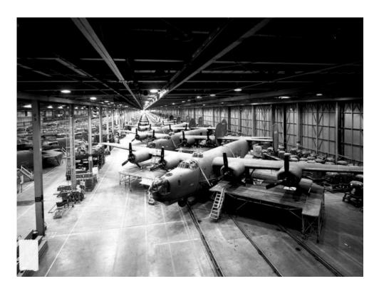
Figure 4.3: General Motor's Willow Run plant, named for the nearby creek, produced one B-24 bomber every hour during WWII. Architect Albert Kahn called this "the largest room in the history of man" (Corps 1940)
