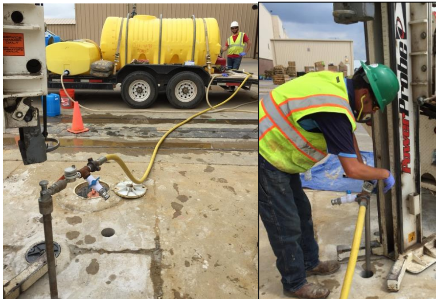
Figure 4.20. Injecting mixed CB1190 culture through direct push rods.
