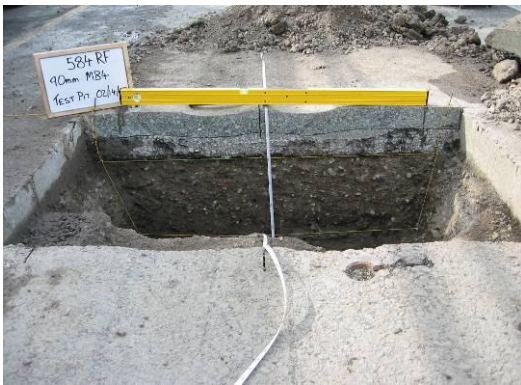
Total view of test pit
