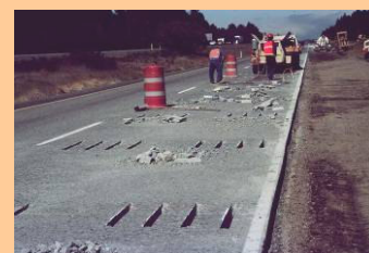
Preventive maintenance - dowel bar retrofit
