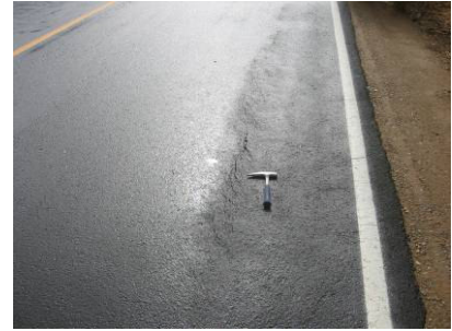
Surface deformation
