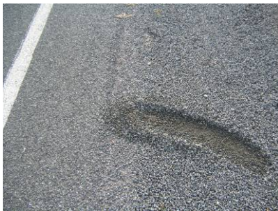
Ravelling from chip seal
