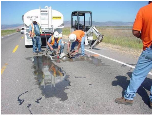
Test pit sawing
