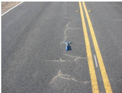
Pumping in new overlay
