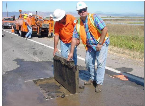
Slab removal
