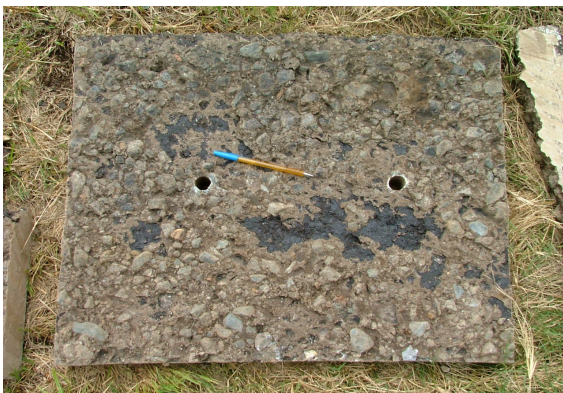
Investigation of slab underside
