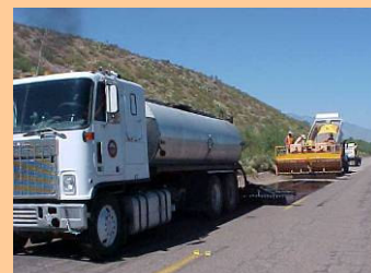
Pavement preservation - chip seal
