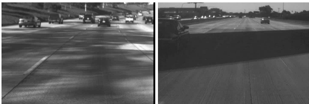
(c) Dark on light lane markings with circular reflectors (d) A combination of segmented lines, circular reflectors, and physical barrier marking lane location
