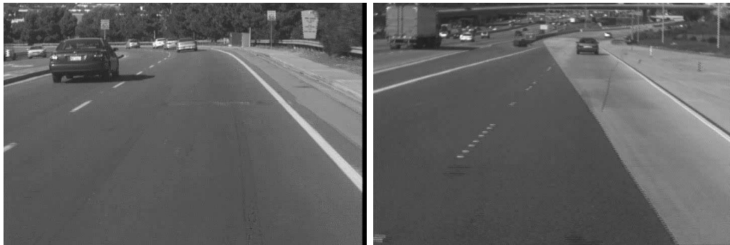
(a) A simple road with solid and segmented line lane markings (b) Circular reflectors and solid-line lane markings with non-uniform pavement texture
