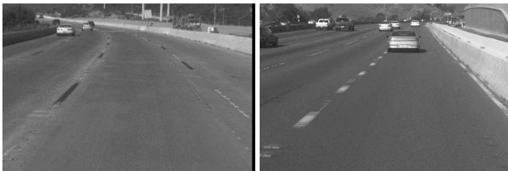
(a) A simple road with solid and segmented line lane markings (b) Circular reflectors and solid-line lane markings with non-uniform pavement texture
